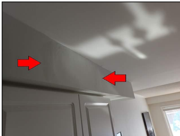
Patched ceiling/bulkhead below Bathroom
