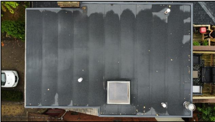
1. Modified bitumen membrane
