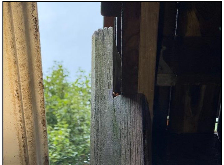
20. Twisted / not fastened to deck
