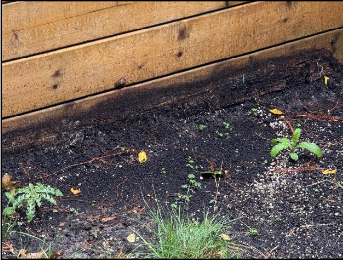
13. wood/soil contact at skirting
