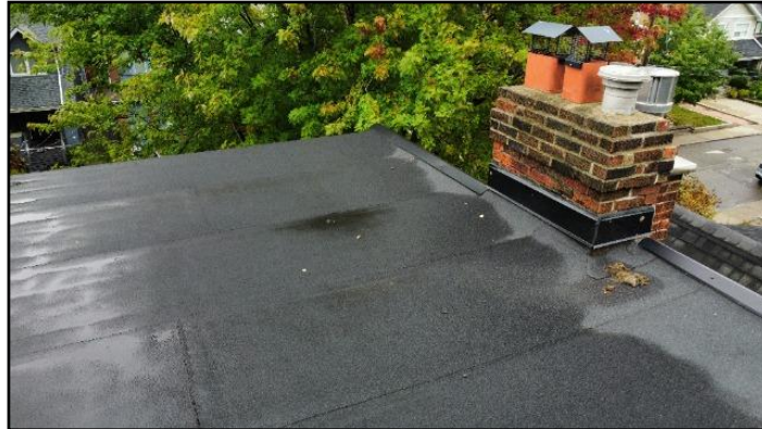
33. No drip edge on cap (crown)
