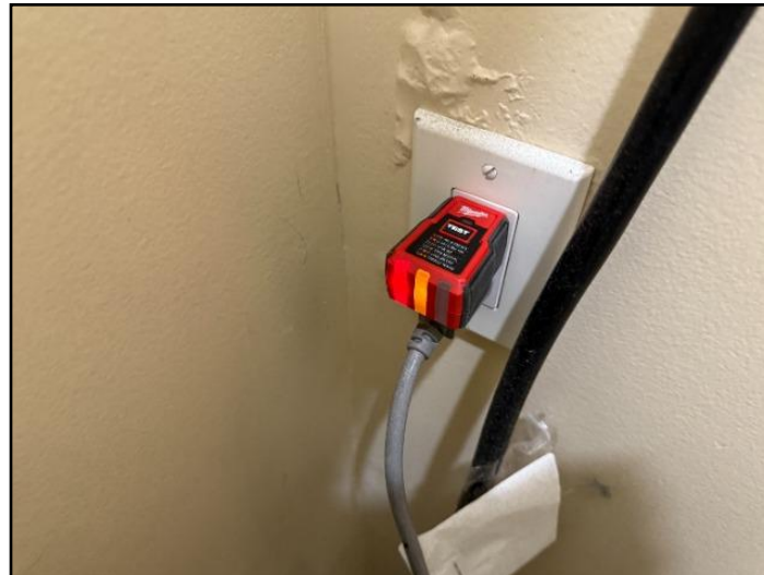
32. Reversed polarity
