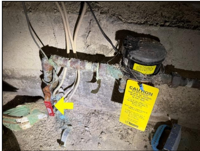
34. Main water shut off valve - Front of the...
