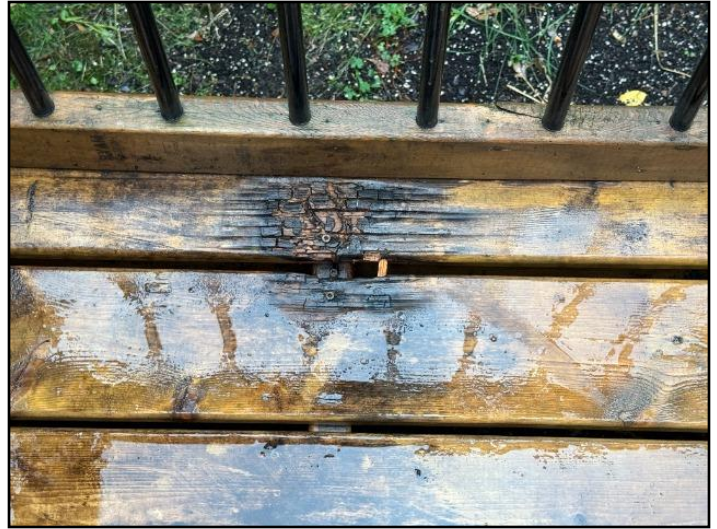
18. Damaged deck board
