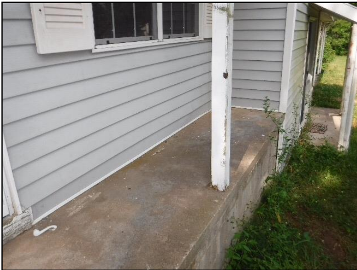
Spindles (balusters) missing
