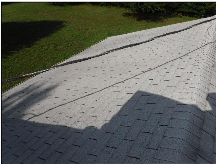
The asphalt shingles on the roof are 3 tab...
