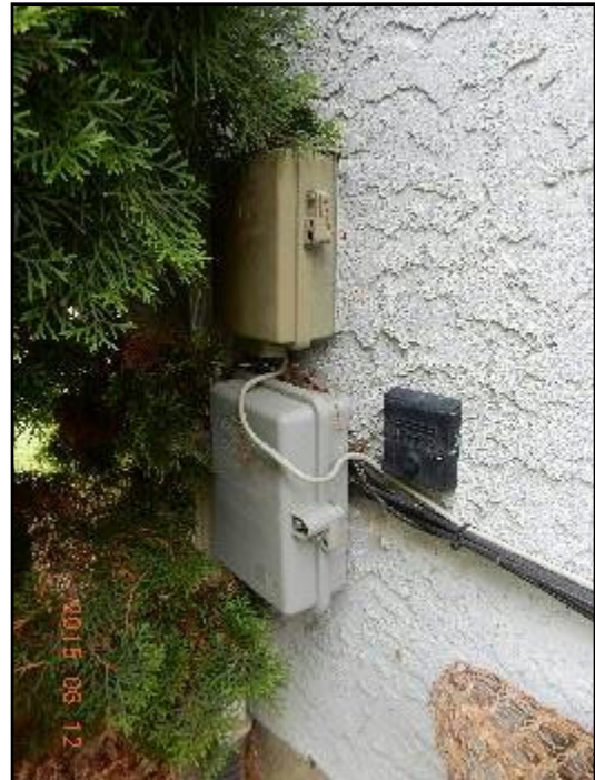
14. Phone + cable + remote water meter
