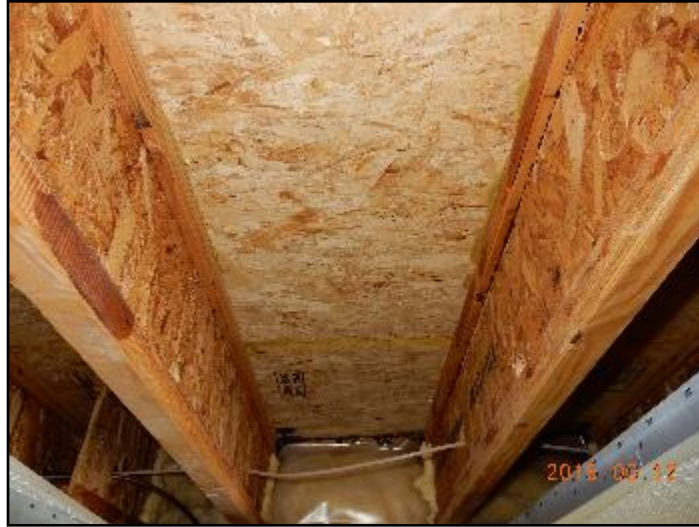
43. OSB subfloor w/ wood I-Joists
