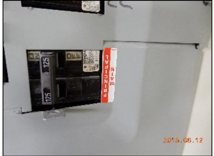
50. 125 amp main electrical disconnect
