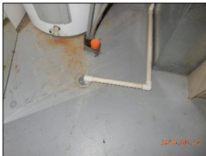
88. Floor drain w/ condensate drain line
