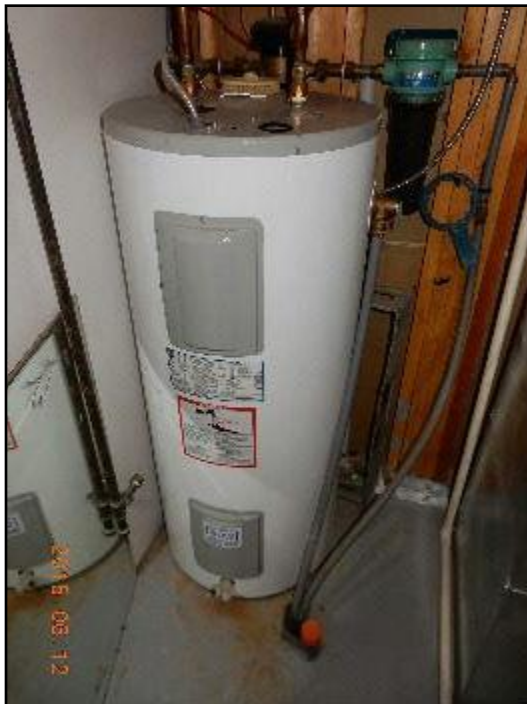
86. Electric hot water heater
