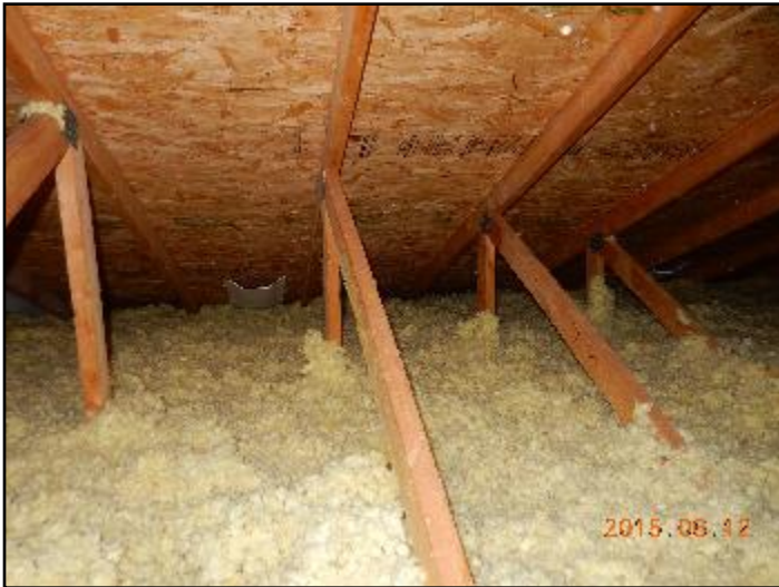
44. OSB roof sheathing
