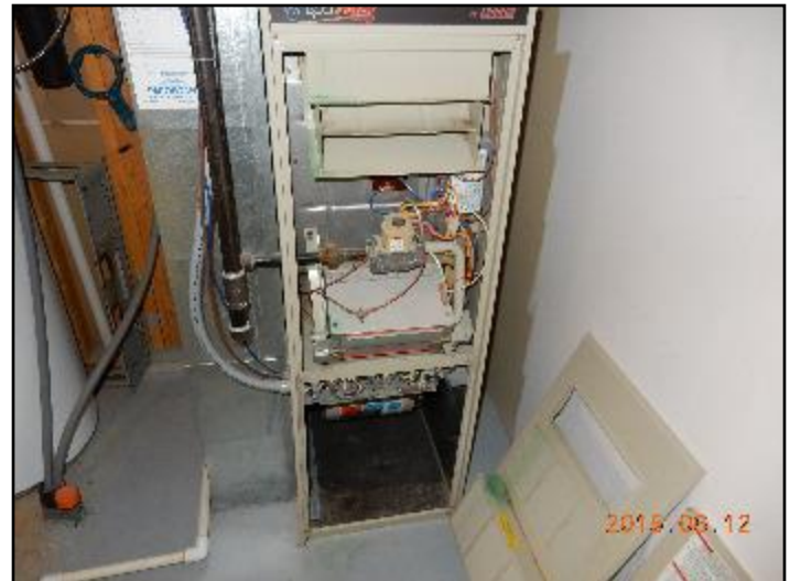
61. Furnace w/ cover removed
