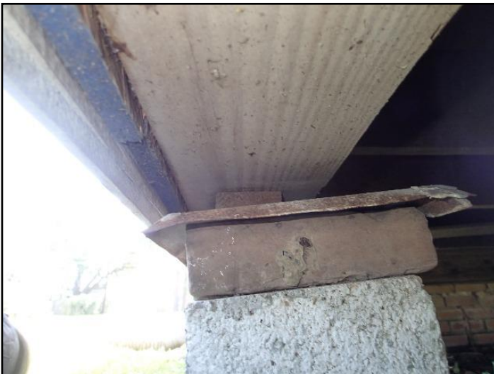
38. Poor bearing
