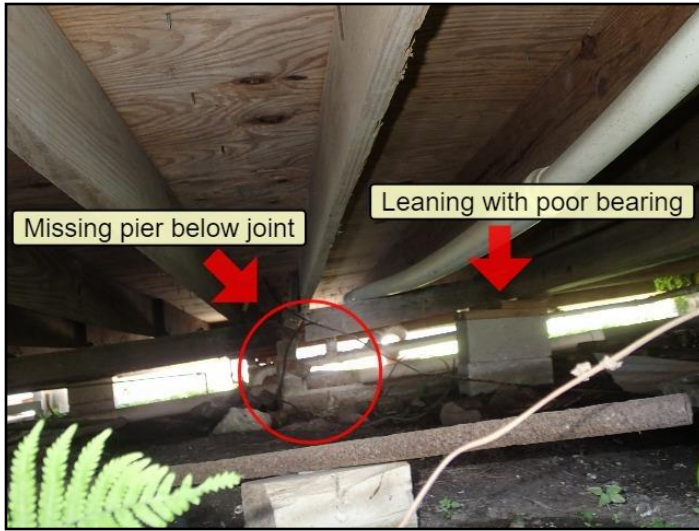
40. Missing pier & leaning pier with poor support
