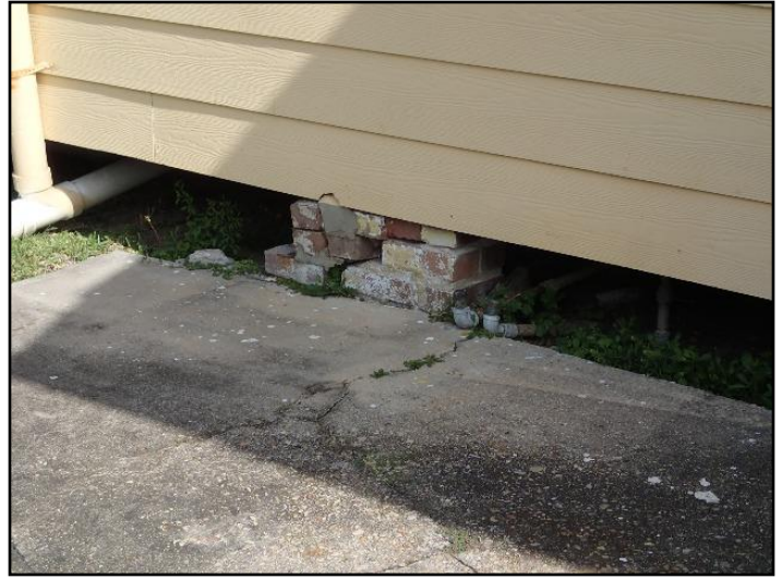
33. Damaged pier
