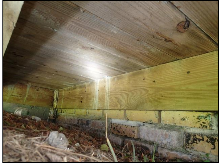
19. Ledger board not properly secured to home
