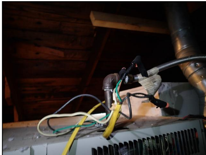
54. No junction box on connection
