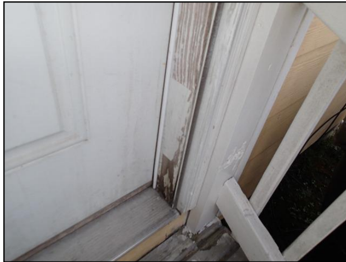
15. Peeling paint, or stain needed on exterior...
