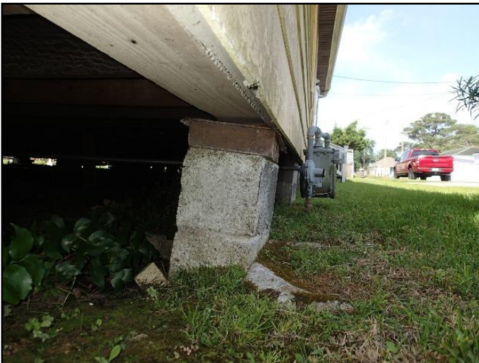
34. Leaning pier with poor support
