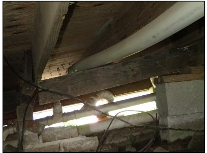
41. Missing pier close up
