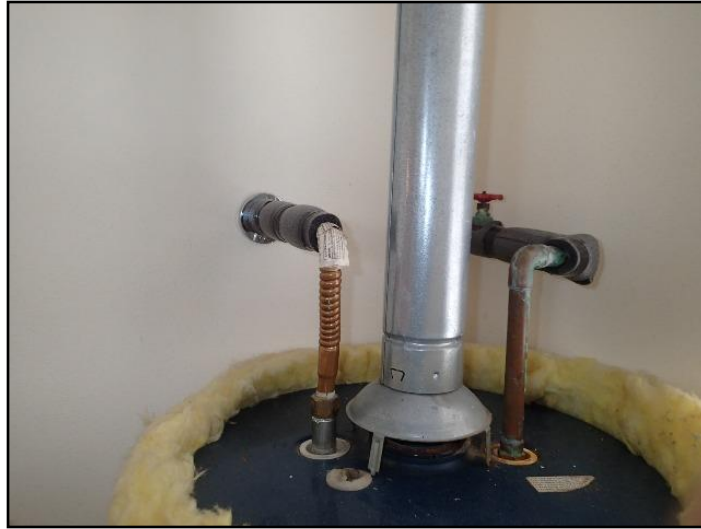
77. Inadequate clearance
