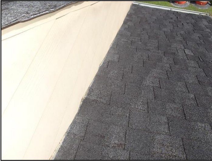
10. No visible flashing and no spacing
