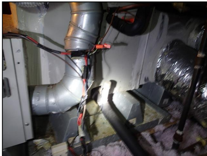
65. Switch in condensate drain line.
