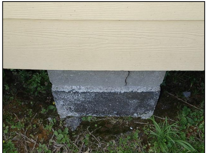
35. Crack in CMU block pier
