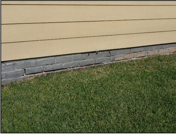
32. Missing mortar
