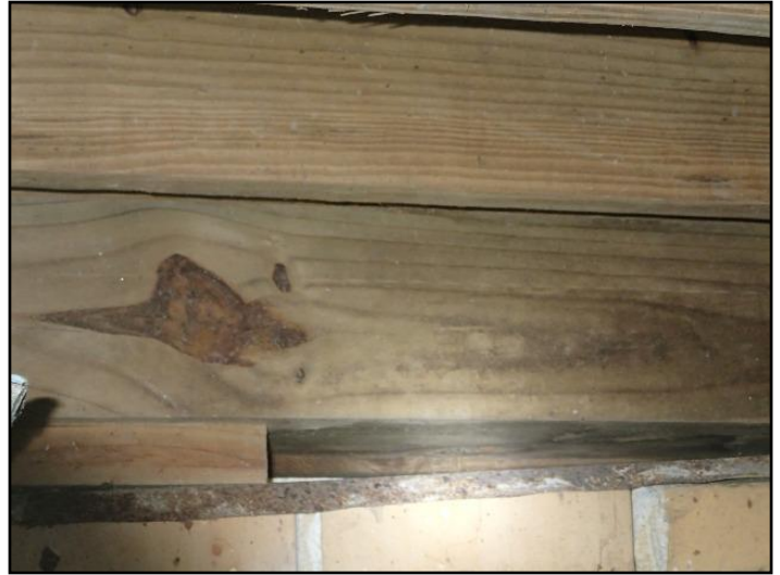
37. Twisted with poor bearing
