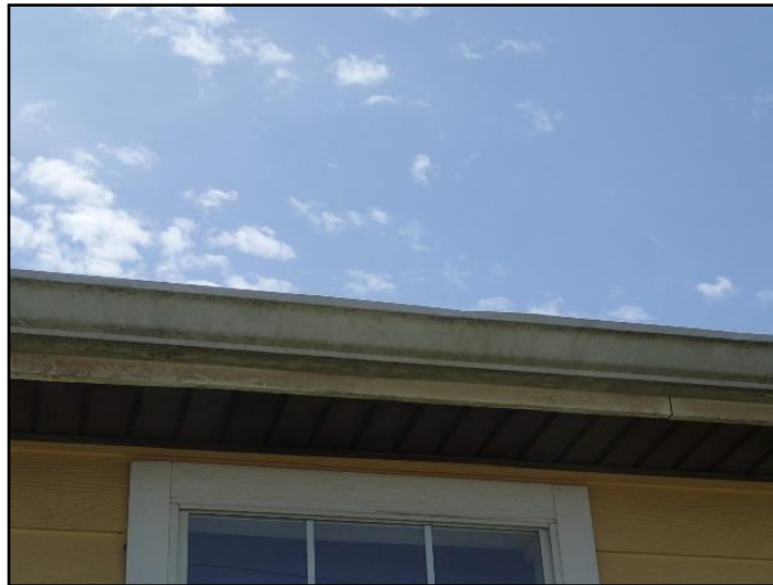
20. Improper slope, ponding
