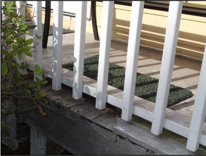
18. Cracked concrete over wood frame
