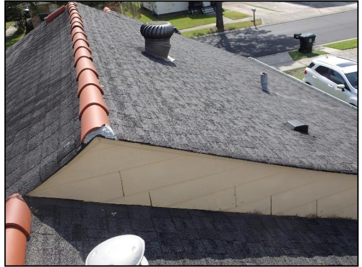
7. No flashing at side wall and granule loss
