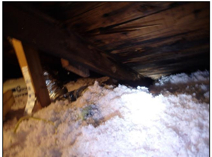
13. Staining on roof decking
