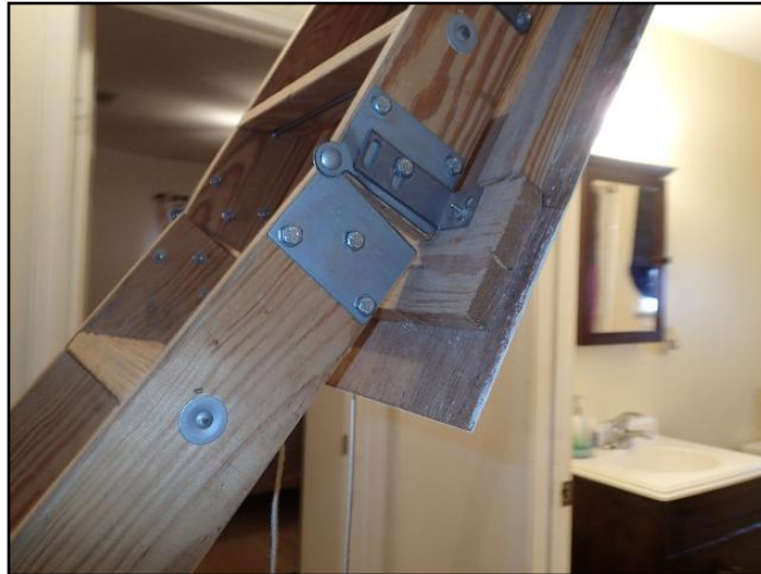
69. Not cut to proper height
