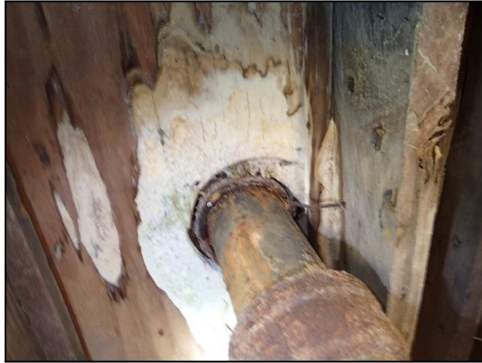
75. Rust at connection and possible split
