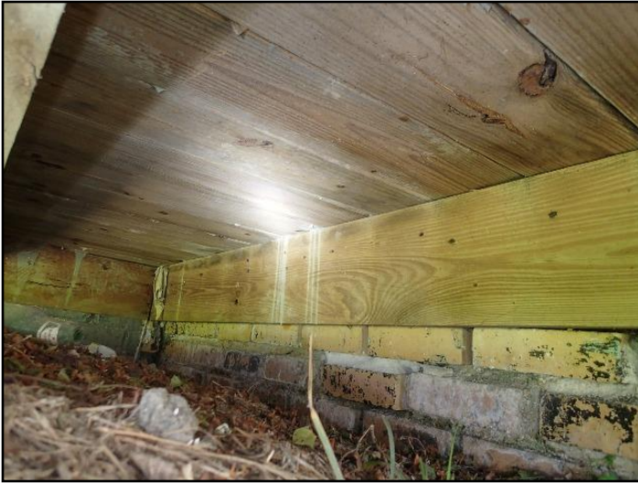
36. Ledger board not connected properly
