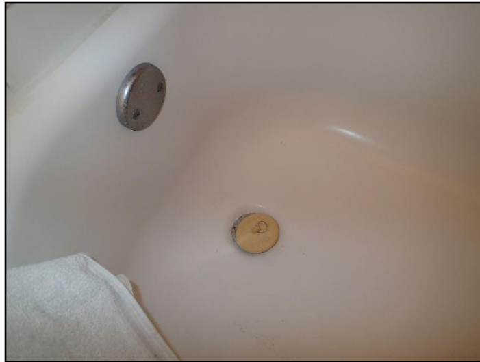
81. Drain stop missing
