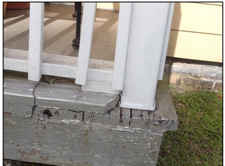
17. Cracked concrete over wood frame
