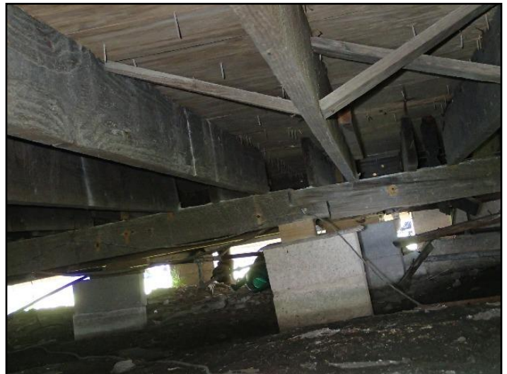
39. Poor bearing below joint
