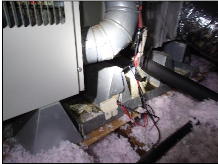
64. Float switch in pan.
