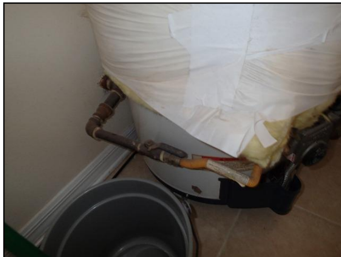
76. Possible wrong type of shut off valve
