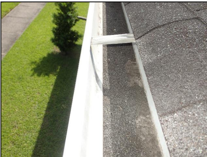
4. Loose granules in gutter
