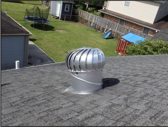
6. Installed at incorrect angle
