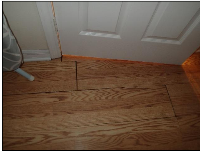
85. Loose or missing sections
