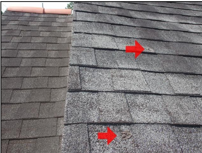
12. Patches/Prior repairs
