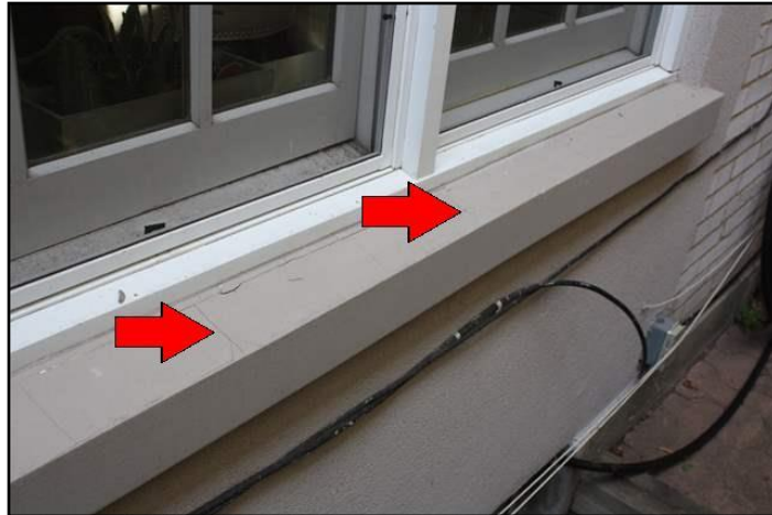
7. small cracks on trim
