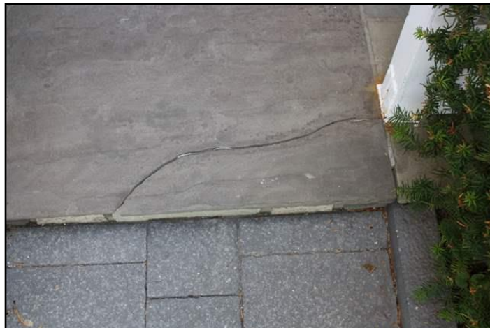
8. Concrete cracked
