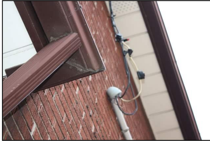
12. Poor connection to service conductors
