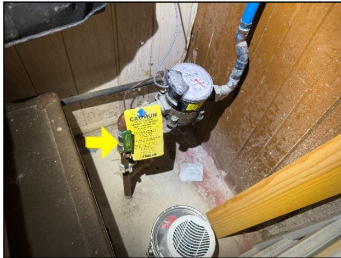
9. Main water shut off valve - Basement
