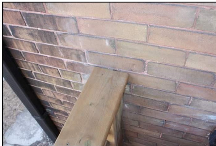
9. Guardrail not secured
