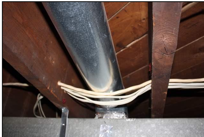
18. Too close to duct, pipe, vent or chimney
