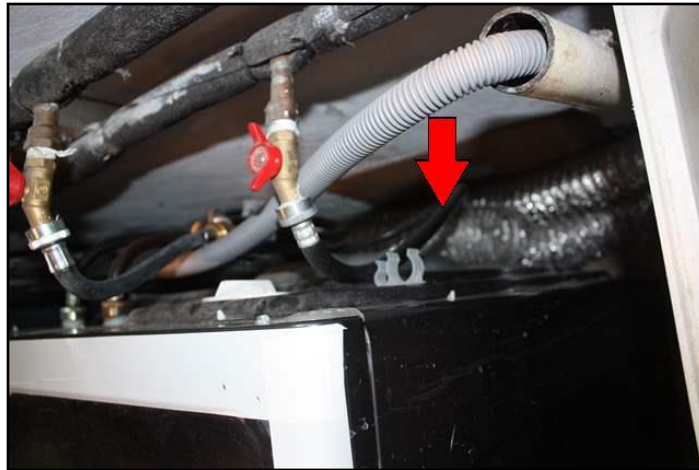
31. Dryer not vented to exterior
