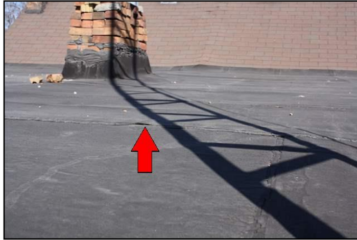
2. Openings at seams or flashings
