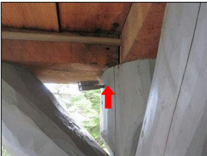
6. Rot in support post not extensive yet
