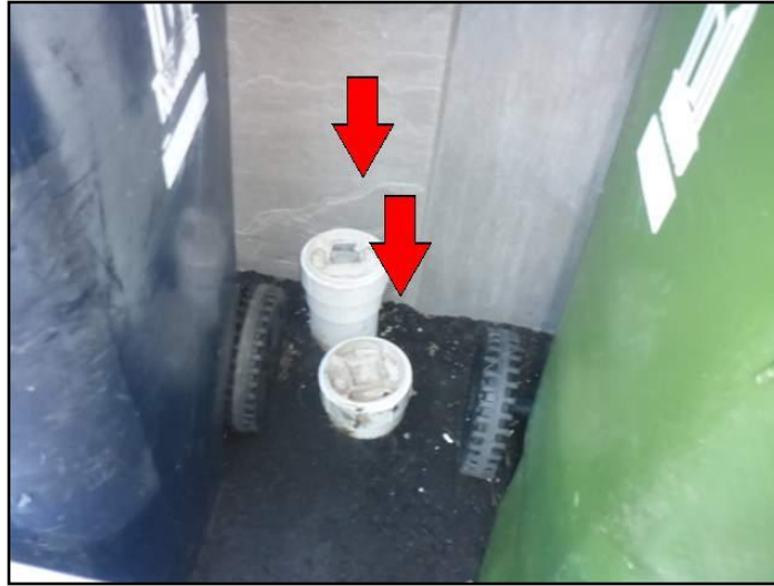
newer cleanouts- drain repairs/upgrades?
