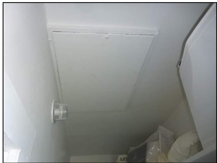
Attic access is difficult
