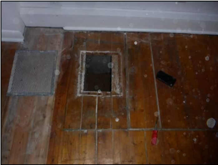
covered pit in rear basement floor
