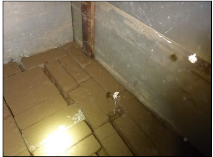
bricks on floor of pit
