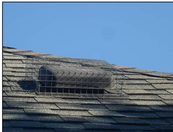
Screen at roof vent
