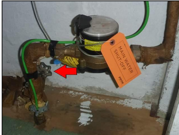
Front of the basement
