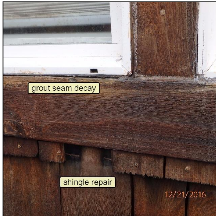
7. Caulking missing or ineffective
