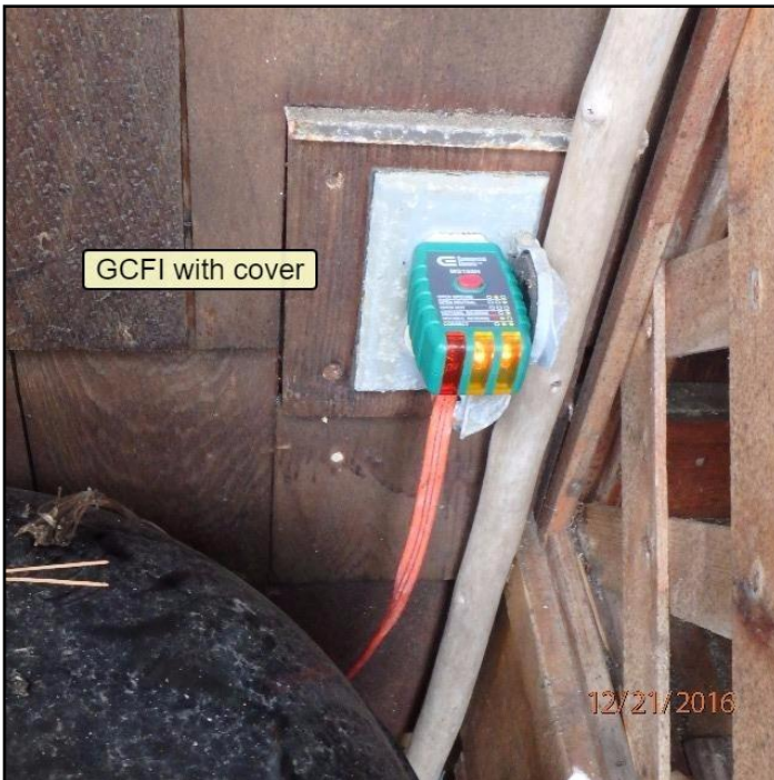
23. No GFCI (Ground Fault Circuit Interrupter)
