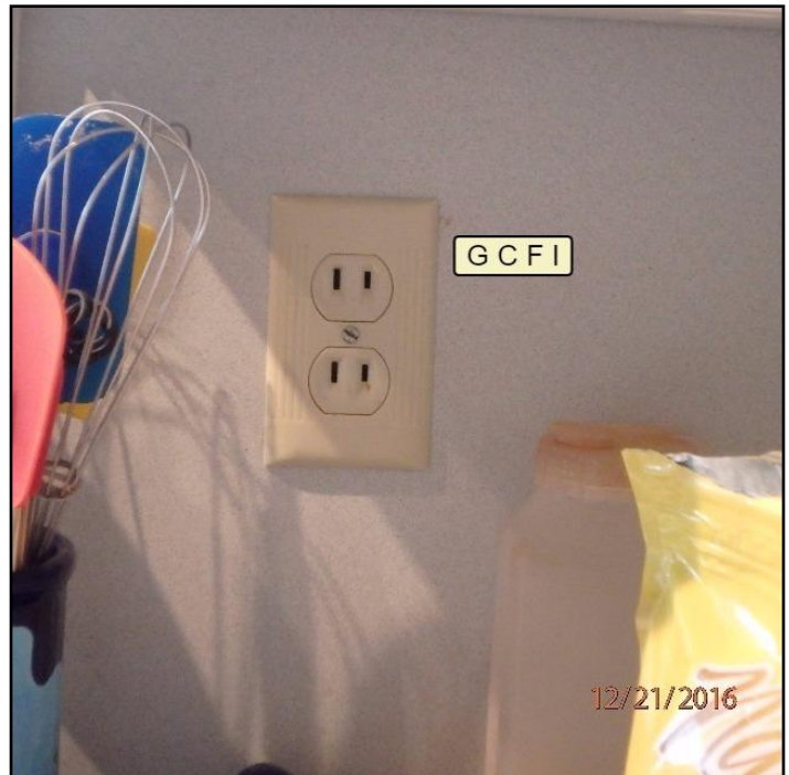
24. No GFCI (Ground Fault Circuit Interrupter)
