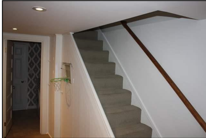
Railing - location incorrect (should be on...
