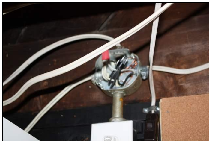
Cover Plate(s) - missing
