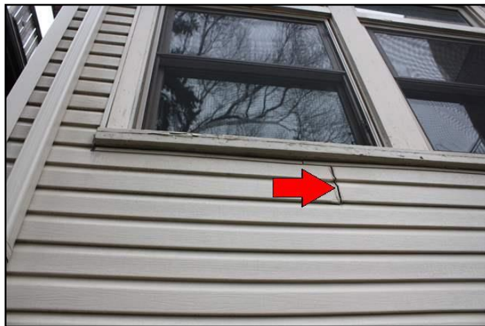
Gap at wall should be sealed
