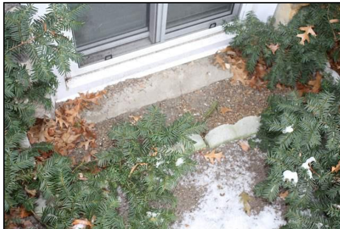
Sill - clearance inadequate (above grade...
