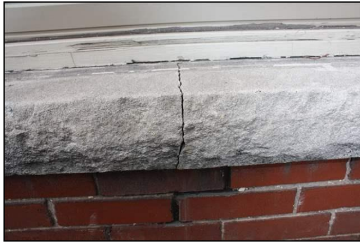
Sill - minor crack
