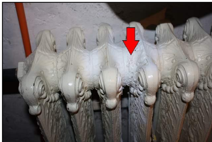
Radiator - leak
