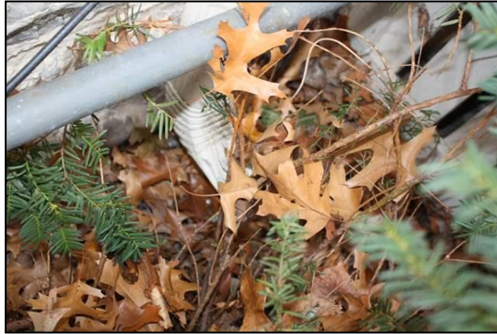
Discharge too close to Foundation (should...
