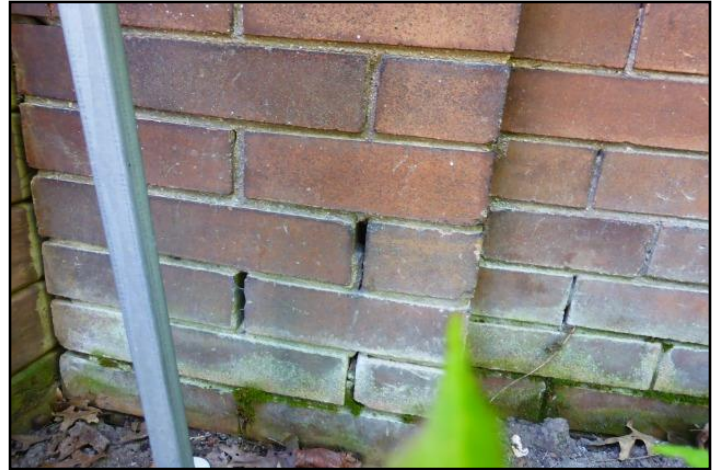
4. Mortar deterioration
