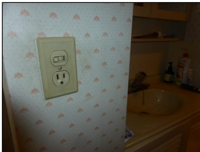
11. GFCI/GFI needed (Ground Fault Circuit...
