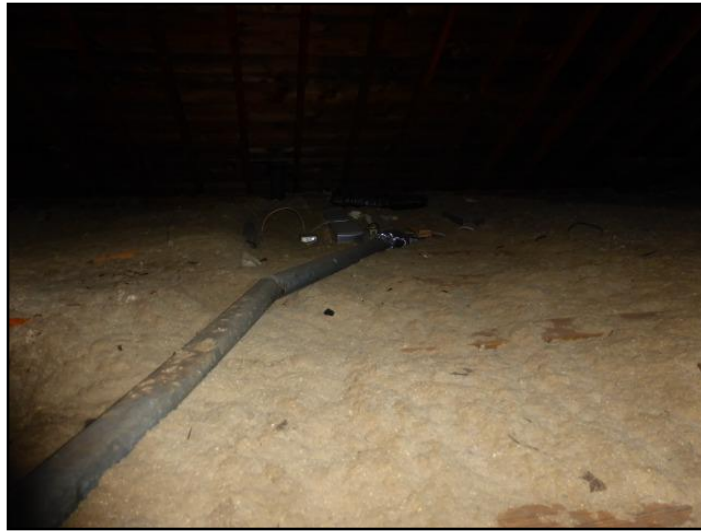
21. Not insulated in unconditioned space
