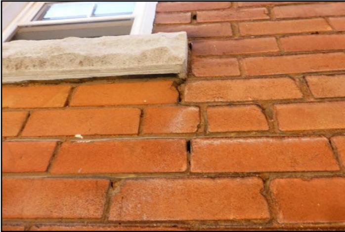
3. Mortar deterioration
