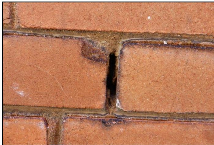
5. Mortar deterioration
