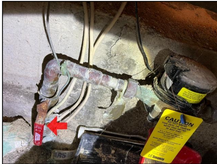
19. main water shut off valve
