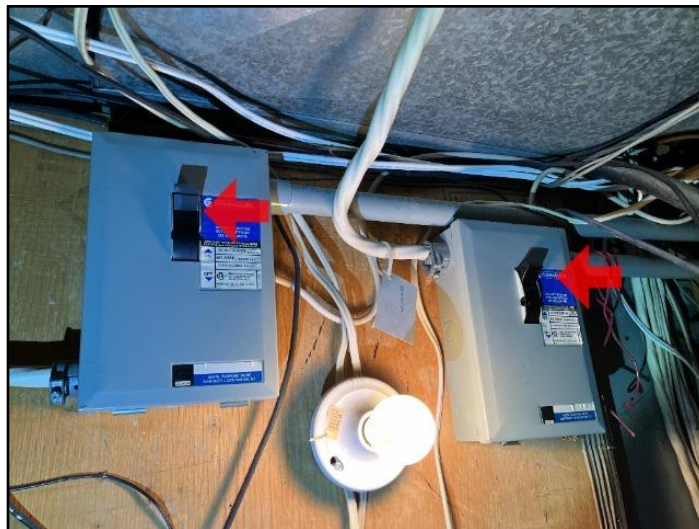
14. Main disconnects for first and third floors
