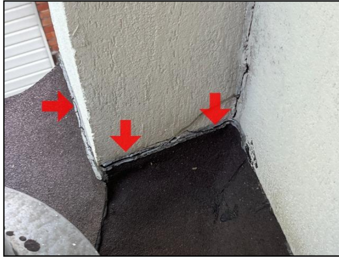
2. Openings at seams or flashings
