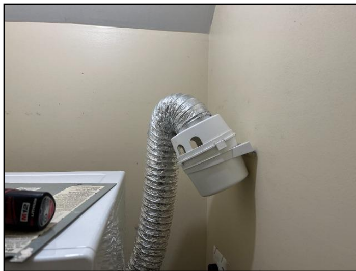
22. Dryer not vented to exterior
