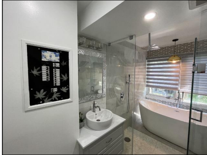
17. Sub panel at bathroom
