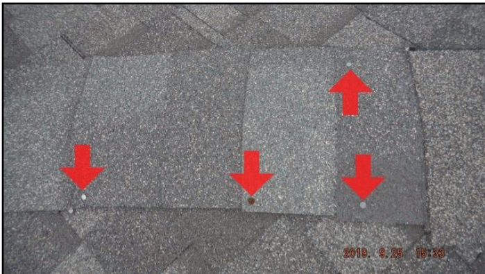
Exposed fasteners
