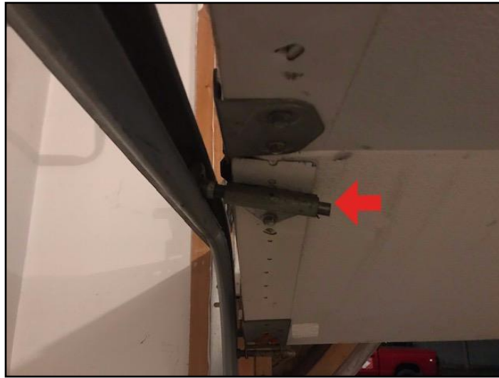
Roller/Panel not attached properly
