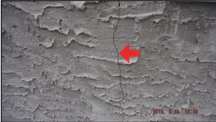
Typical minor cracks
