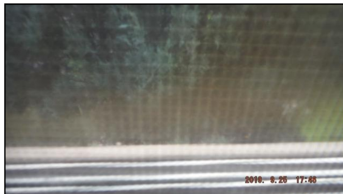
Lost seal on double or triple glazing
