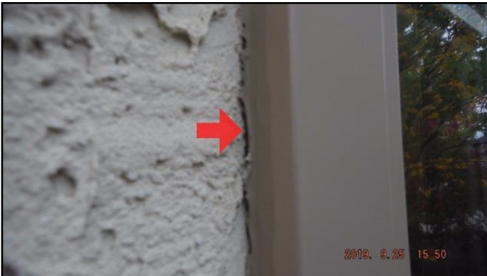
Caulking missing or ineffective
