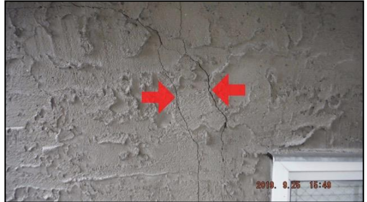
Typical minor cracks
