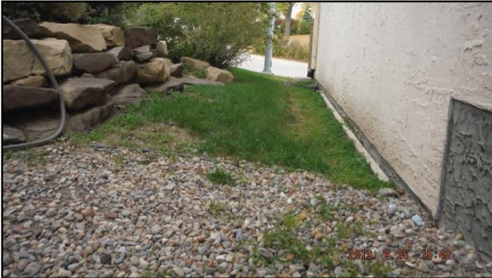
Improper slope or drainage
