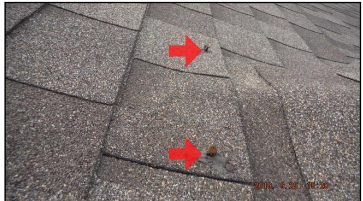
Exposed fasteners
