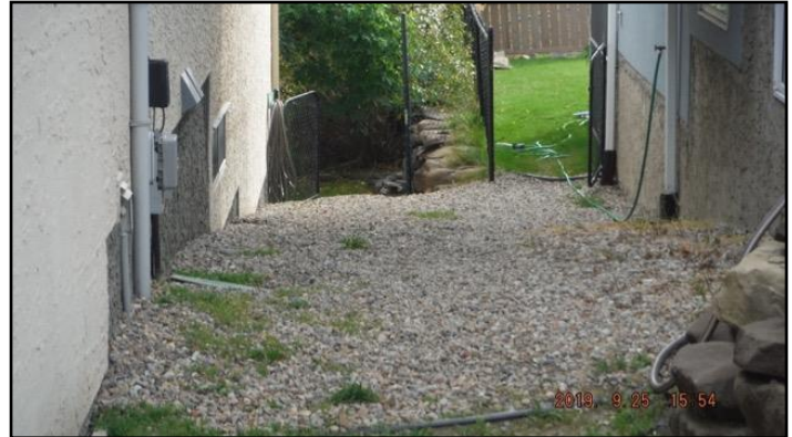
Improper slope or drainage
