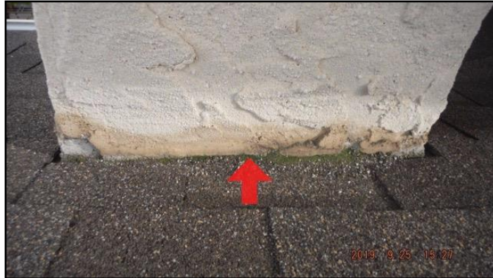
Pan missing, inappropriate
