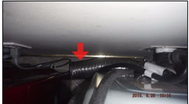
Dryer vent disconnected
