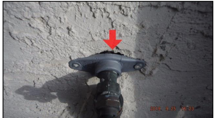
Caulking missing or ineffective
