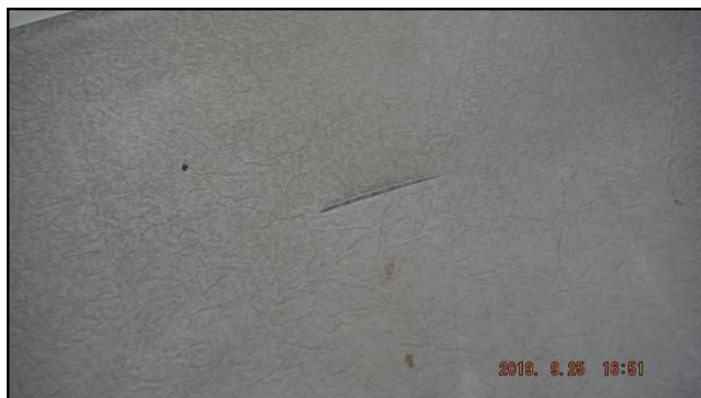
Damaged membrane
