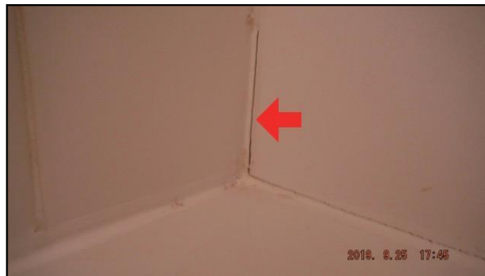
Caulking loose, missing or deteriorated
