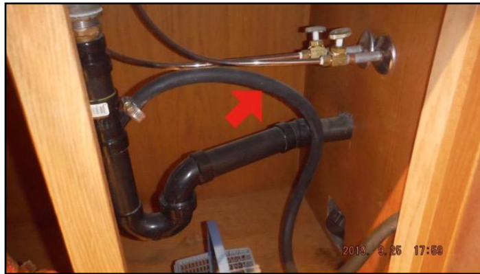
Backflow prevention missing
