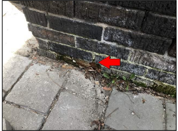
7. Spalling
