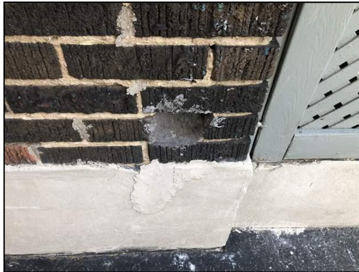
22. Masonry missing
