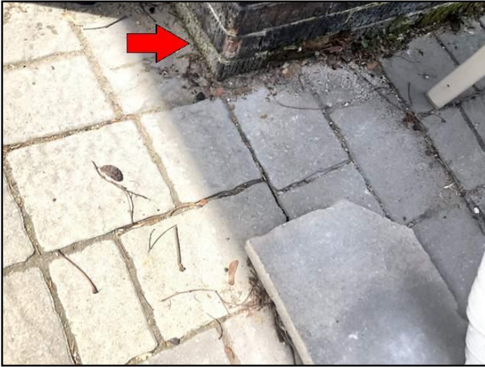
6. Spalling
