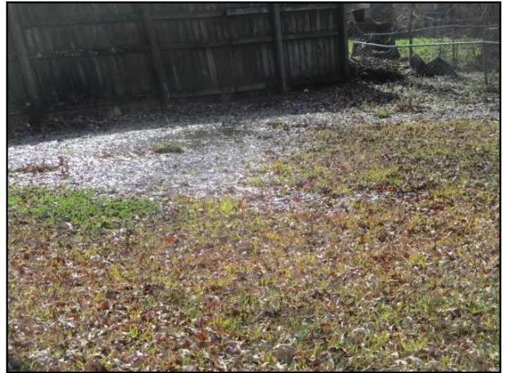
10. Rear grading (ponding)
