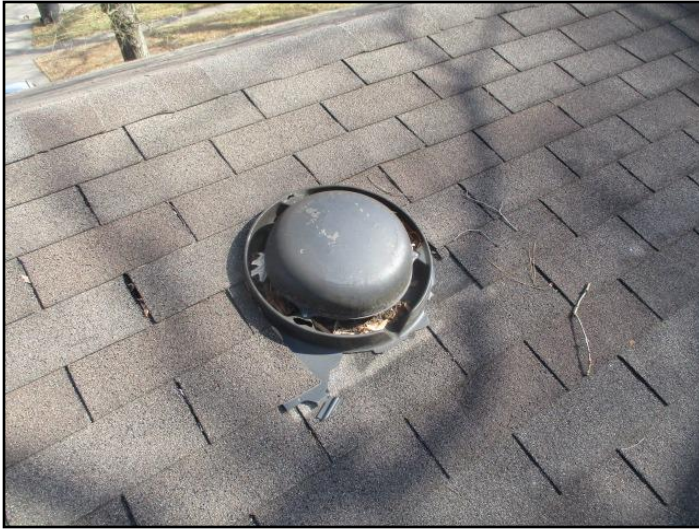
26. Damage roof vent
