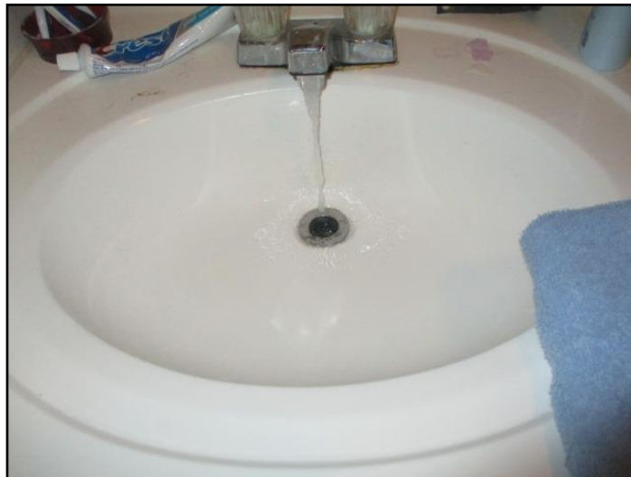
31. Drain stop missing
