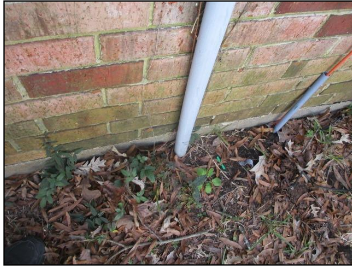
20. Missing ground rod
