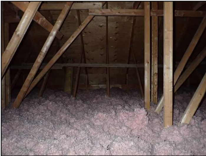
Insulation is evenly distributed
