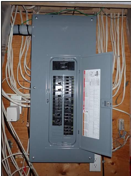
Panel and wiring are in good condition
