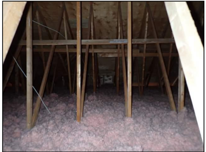
Insulation is evenly distributed
