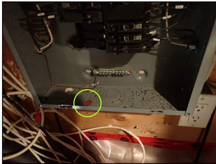
Seal openings in panel
