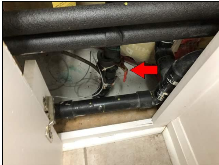
19. Water main shut off valve
