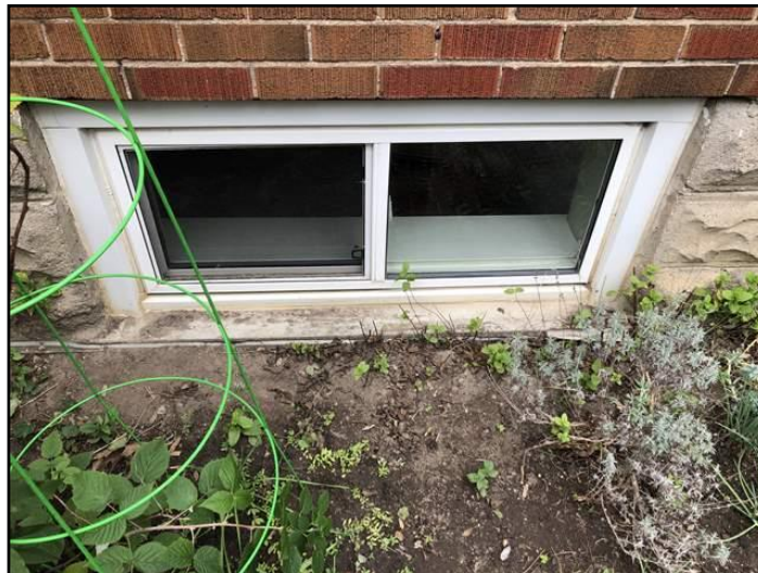
11. Sill - Near or at Grade Level
