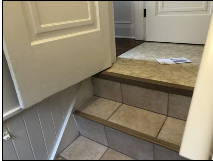
23. Installed backwards
