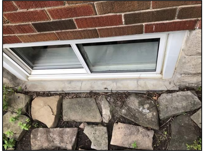
10. Sill - Near or at Grade Level
