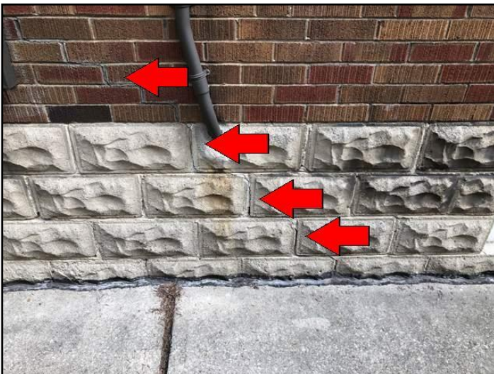
7. Example of typical minor cracks
