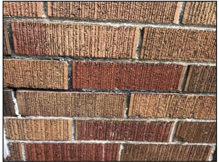
6. Minor mortar deterioration
