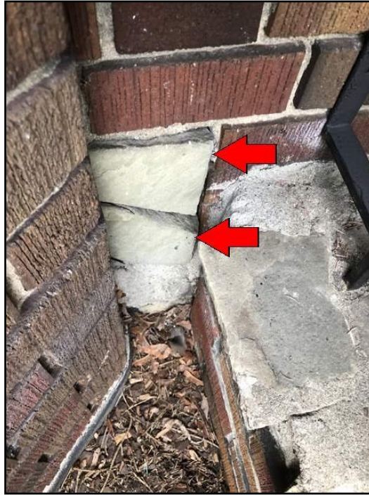
14. Loose masonry
