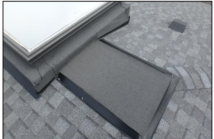
Ex. Modified bitumen membrane
