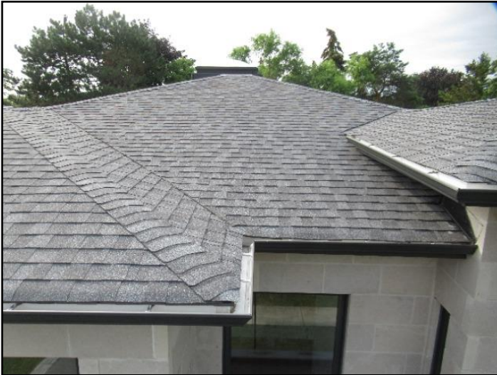
Ex. Architectural/Composition Shingles
