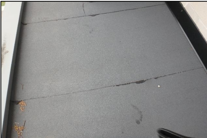
Ex. Modified bitumen membrane
