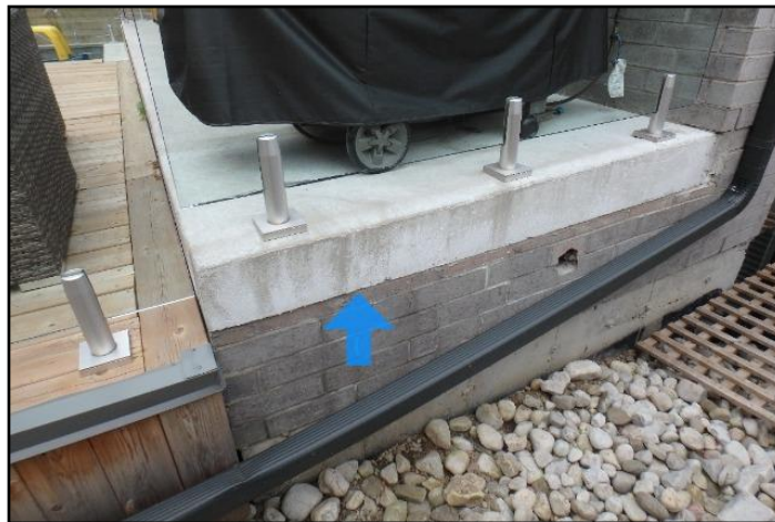
Ex. Drip edge missing/incomplete
