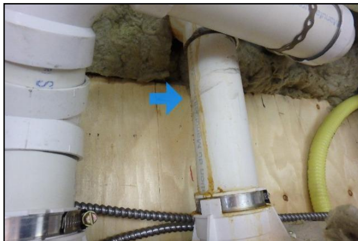
Ex. Evidence of prior leak - dry
