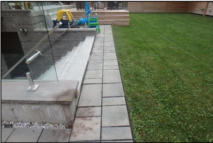
Ex. Grading slopes down toward house
