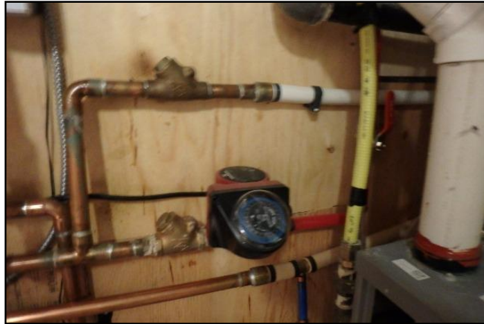
Ex. Circulating pump
