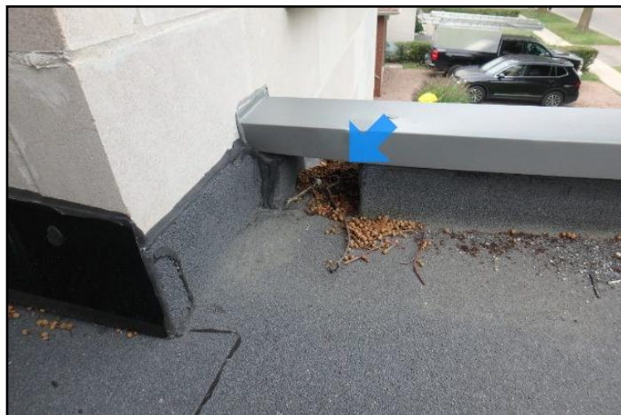
Ex. Flat roof drain
