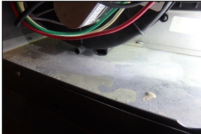
Evidence of past leakage was observed.
