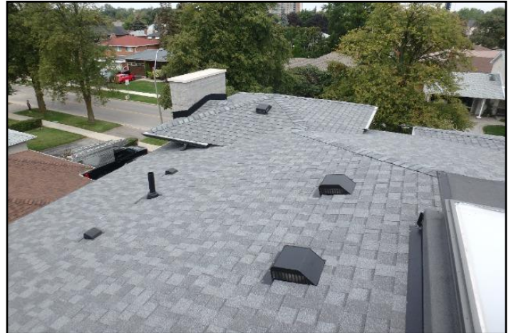
Ex. Architectural/Composition Shingles
