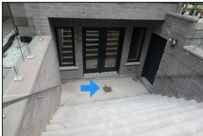
Drains missing, clogged or undersized
