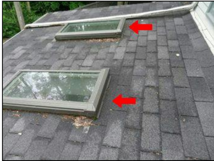
proper installation of skylight.
