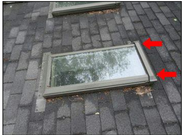
proper installation of skylight.
