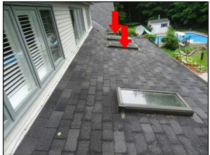
proper installation of skylight.
