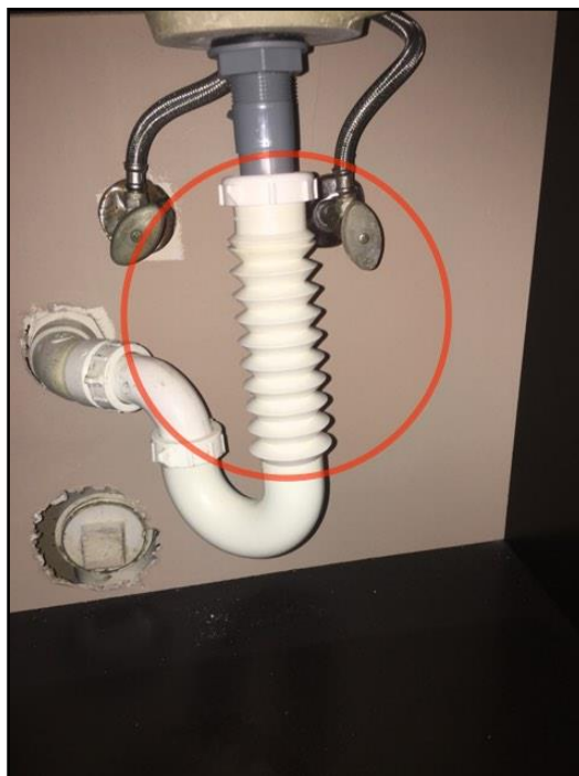
98. Corrugated piping is not ridged nor...
