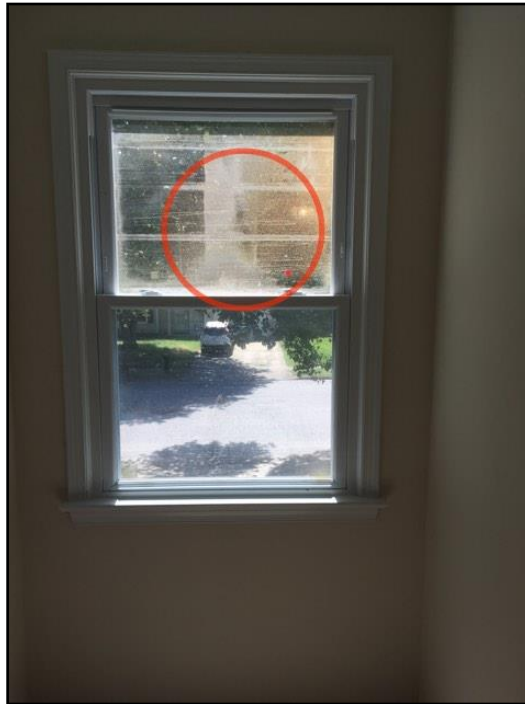
106. Lost seal on double or triple glazing
