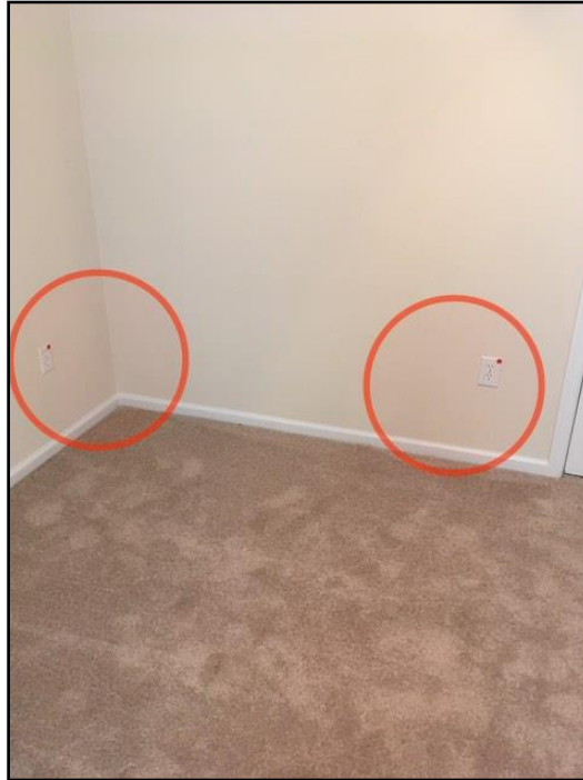
26. Reversed polarity
