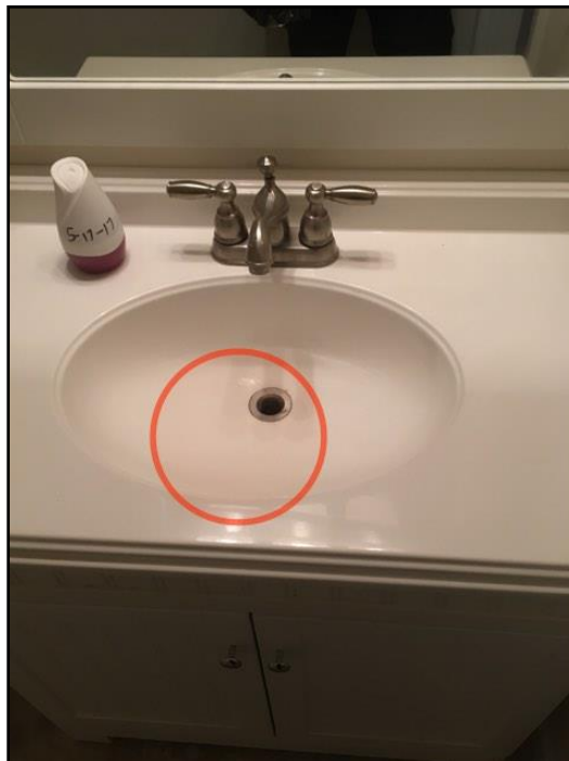
32. Drain stop missing
