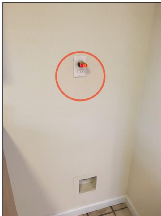
79. Reversed polarity
