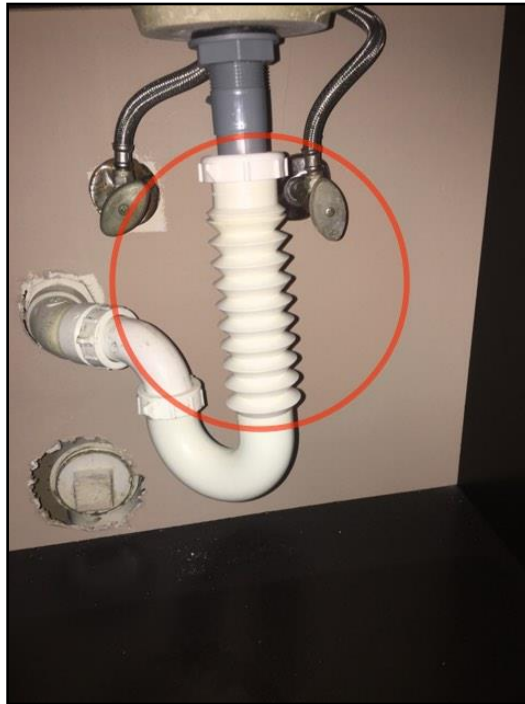
31. Corrugated piping is not ridged nor...
