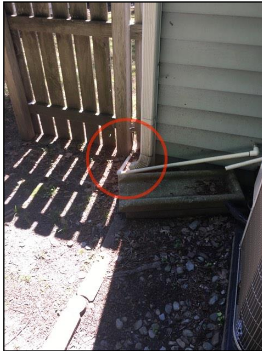
52. Should discharge 6 feet from building
