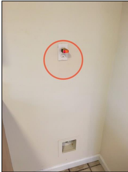
24. Reversed polarity
