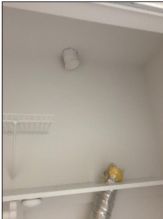
111. Dryer vent disconnected
