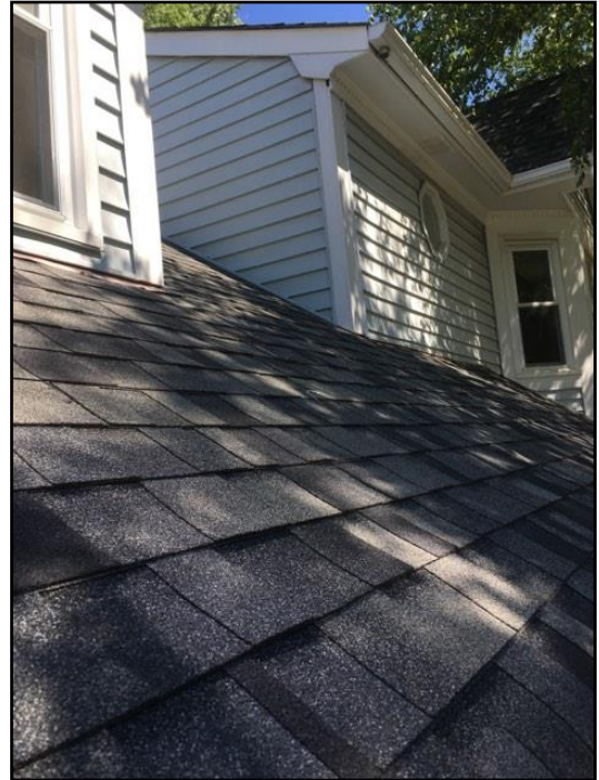
43. Architectural Asphalt Shingles typical life...
