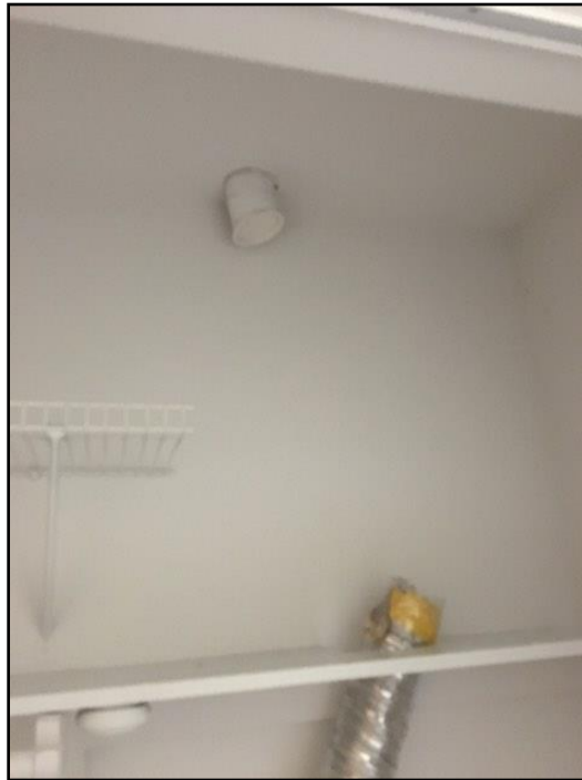
41. Dryer vent disconnected
