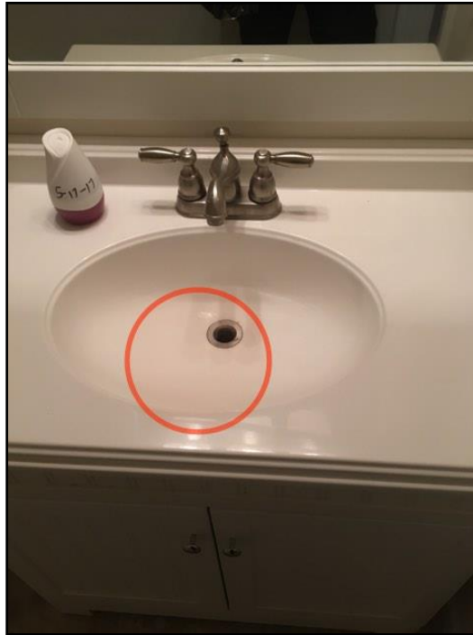
99. Drain stop missing
