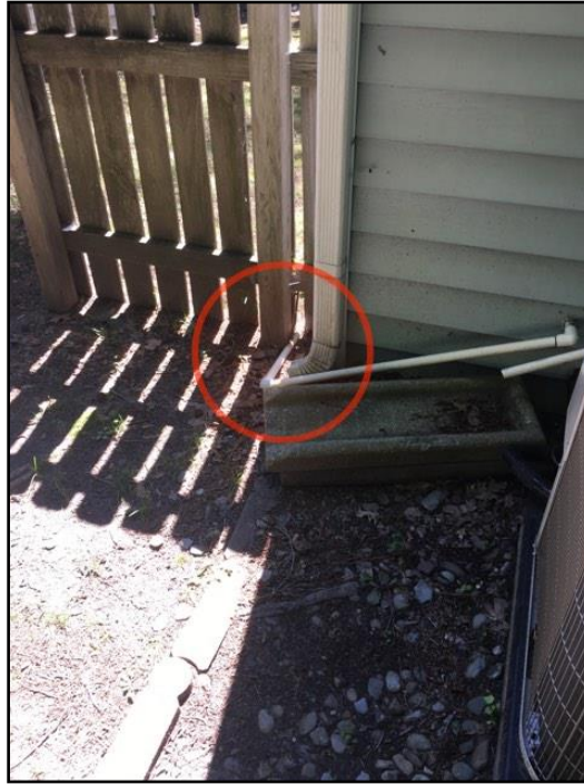
5. Should discharge 6 feet from building
