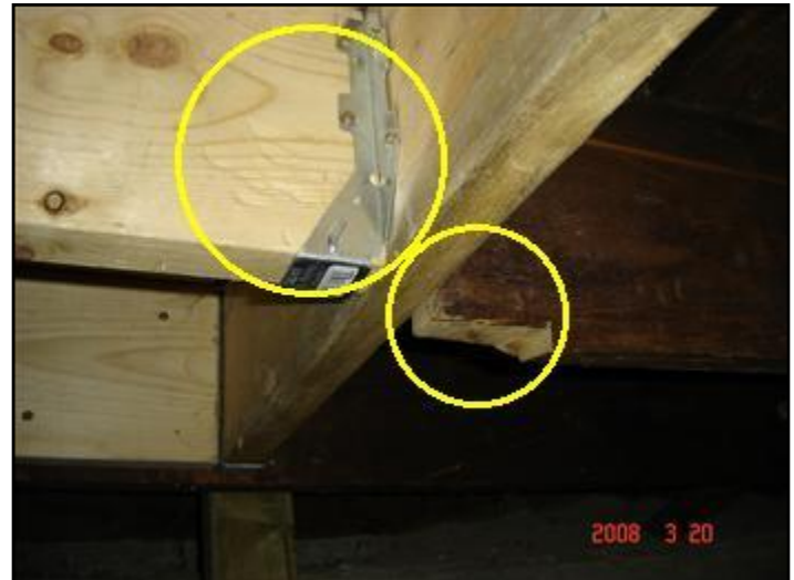
on side of beam with joist hangers
