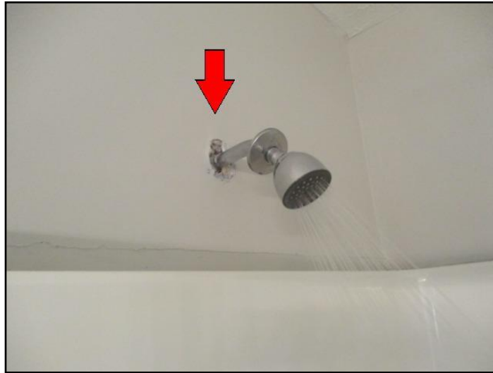
Caulking loose, missing or deteriorated
