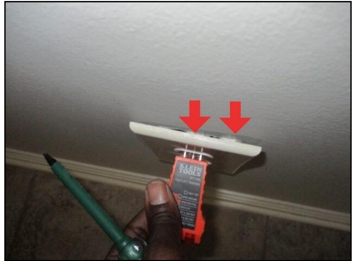
For outlet (receptacle) is loose
