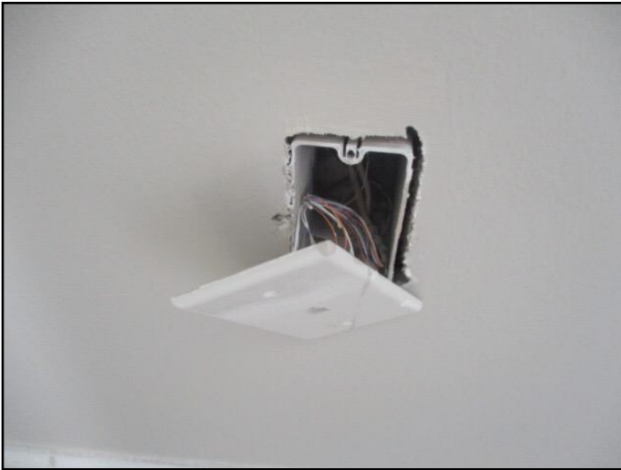
For outlet (receptacle) is loose
