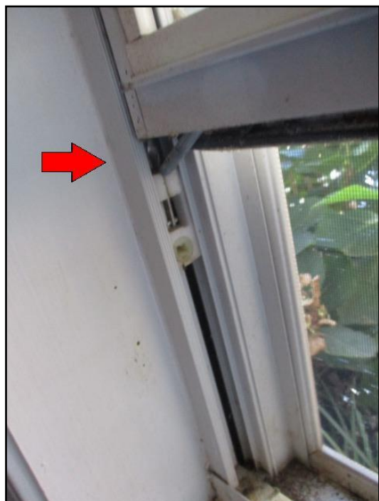
Broken sash and spring
