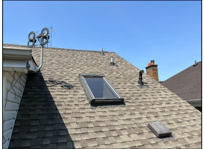
2. Asphalt shingles
