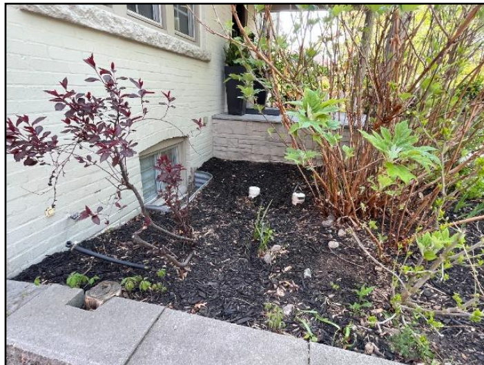
12. Improper slope or drainage
