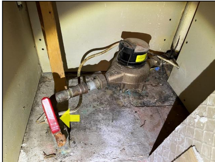
20. Main water shut off valve
