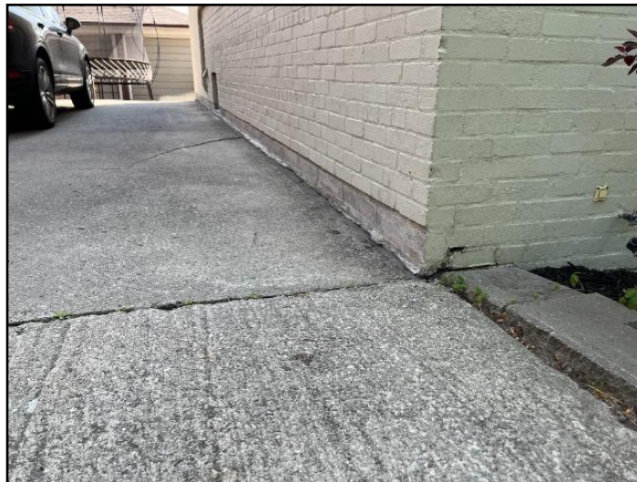
13. Improper slope or drainage
