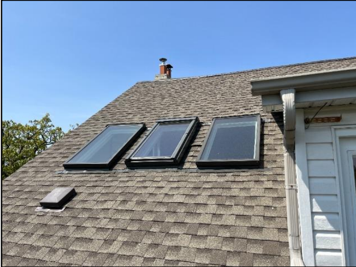
1. Asphalt shingles
