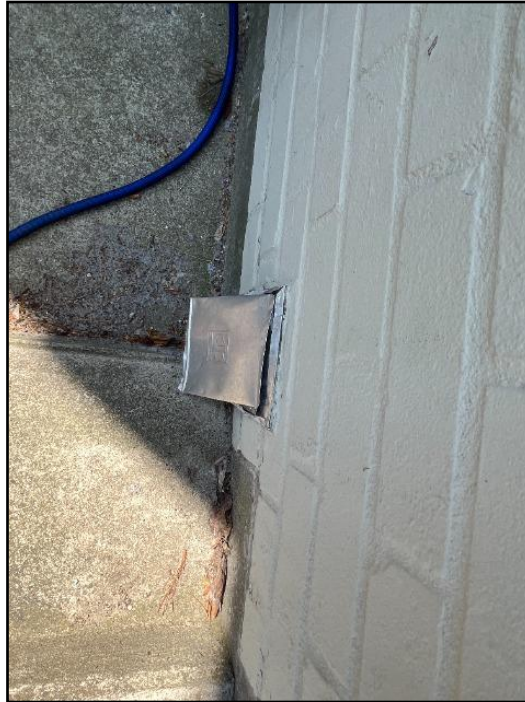
3. Caulking missing or ineffective
