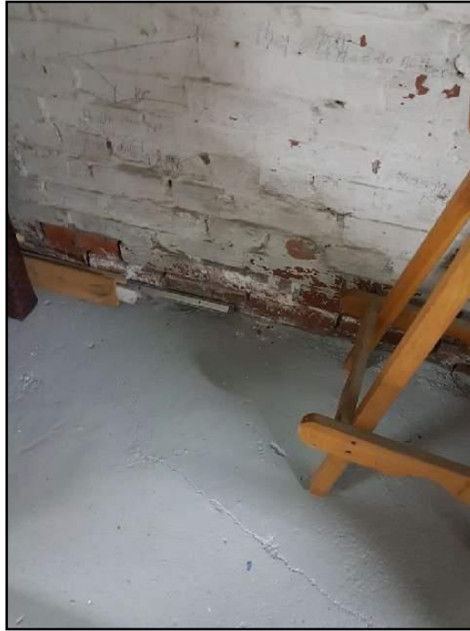
18. Efflorescence
