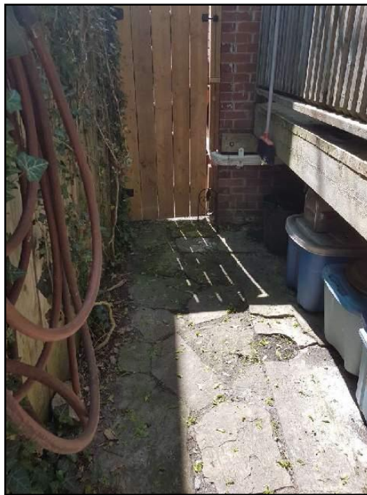
4. Improper slope or drainage
