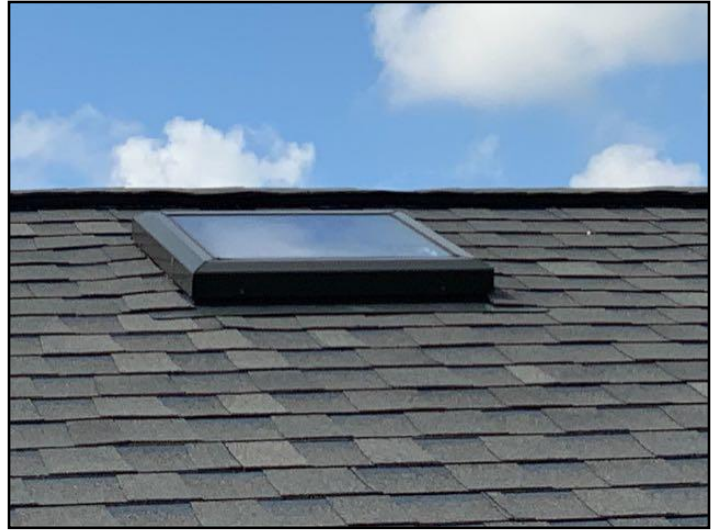
11. Skylight not well secured
