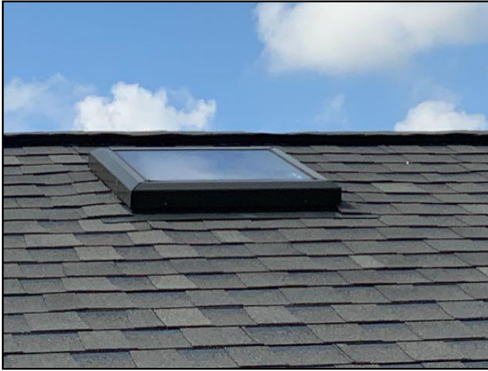
10. Skylight not well secured
