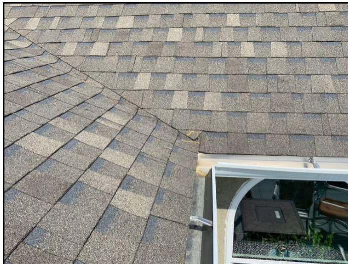
9. Exposed fasteners
