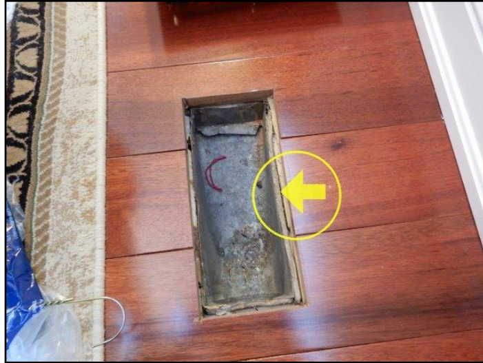
42. Possible asbestos containing materials
