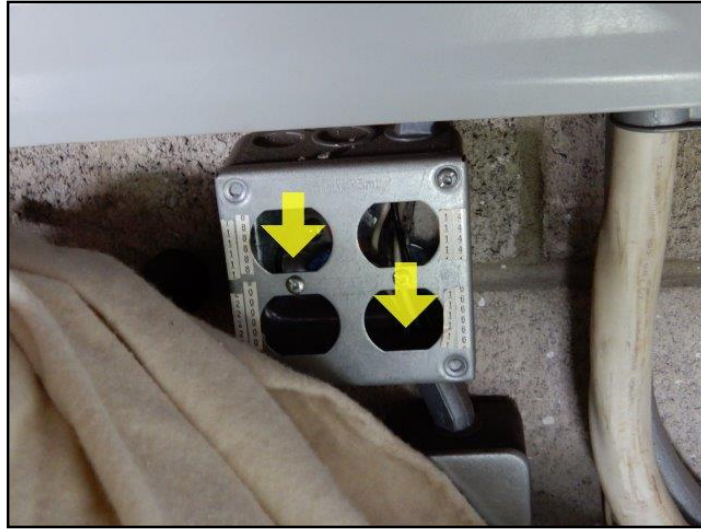
21. Unprotected openings
