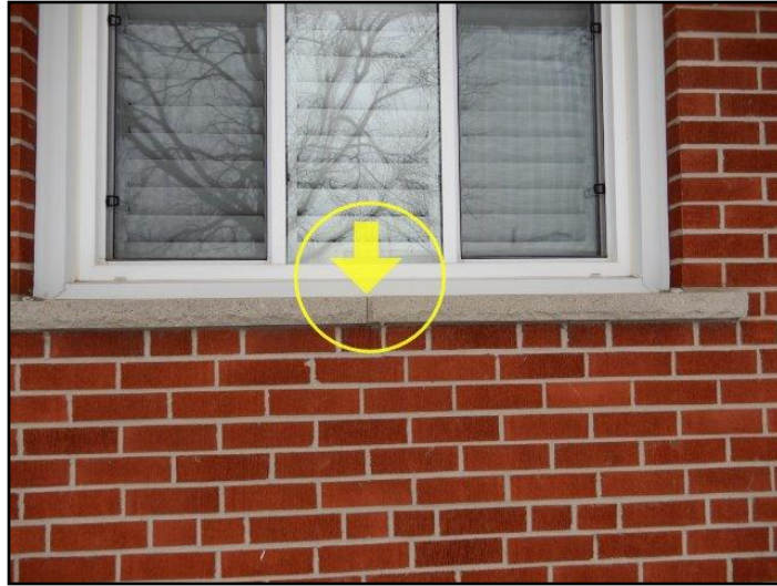
7. Caulking loose, missing or deteriorated
