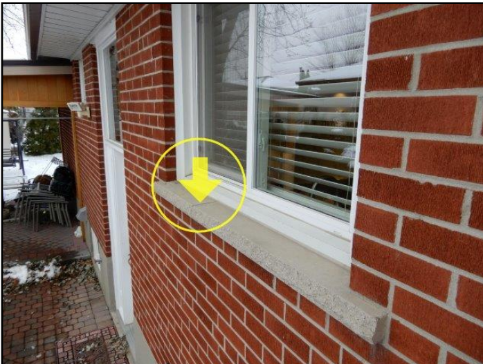
5. Caulking loose, missing or deteriorated
