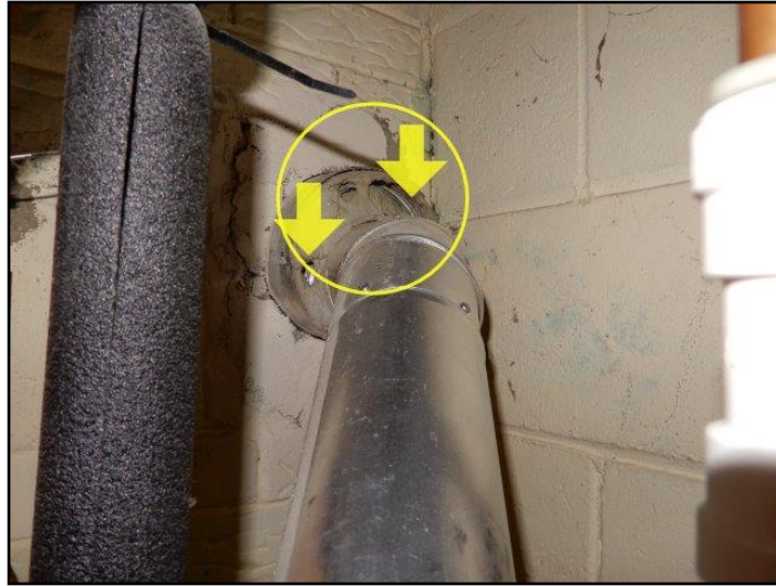
37. Poor connections
