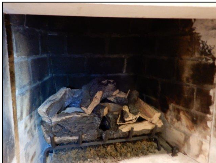
33. Damper in existing fireplace not fixed open
