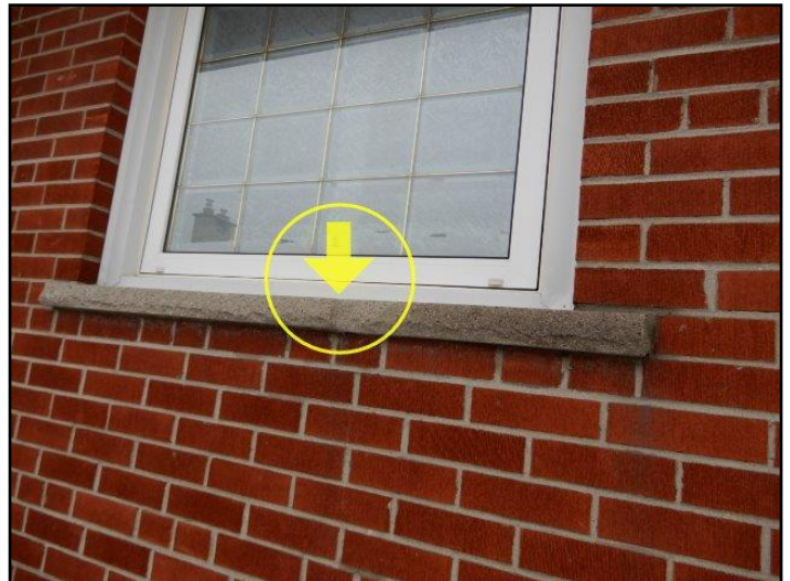
6. Caulking loose, missing or deteriorated
