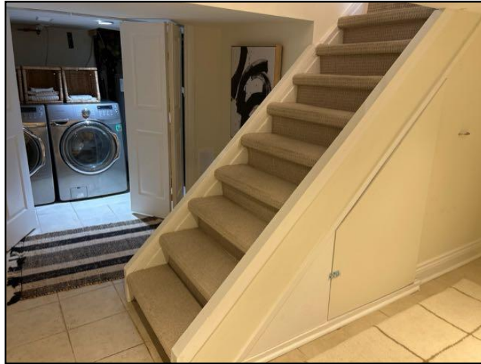
Missing handrail/guard
