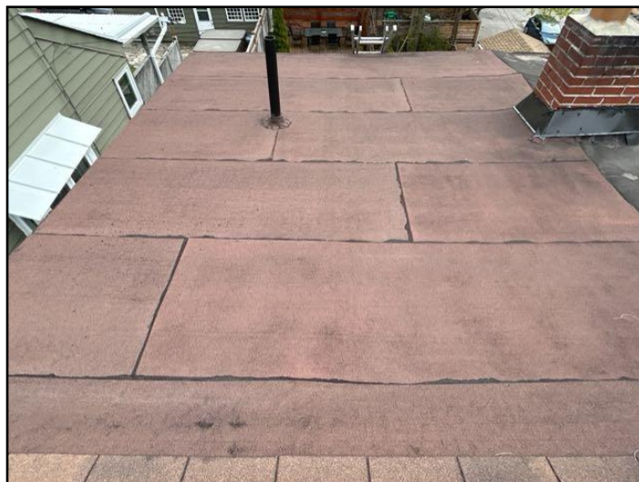
Modified bitumen membrane
