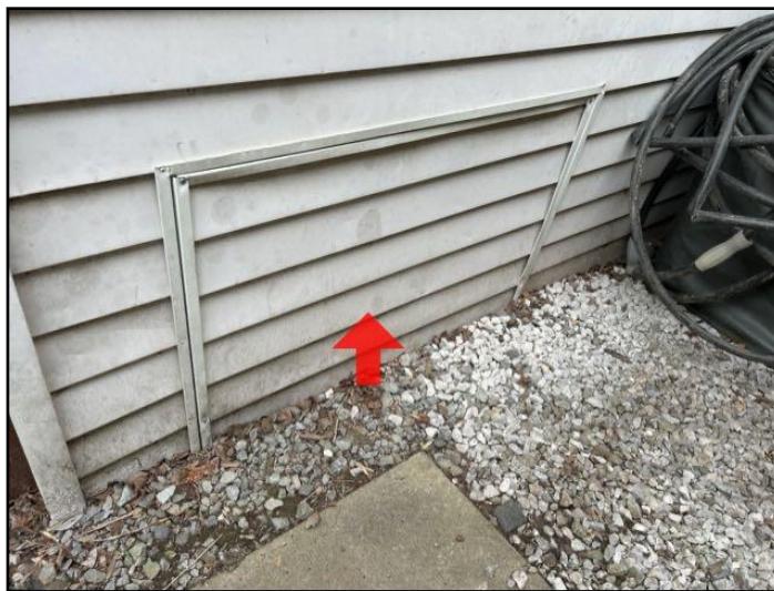
Crawlspace access hatch
