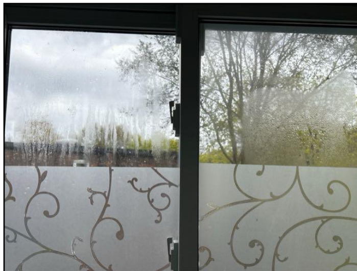
Lost seal on double or triple glazing
