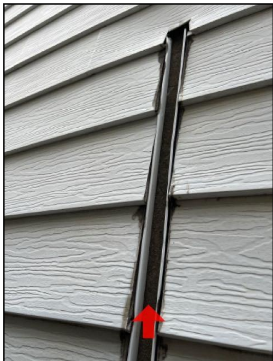
Abandoned raceway
