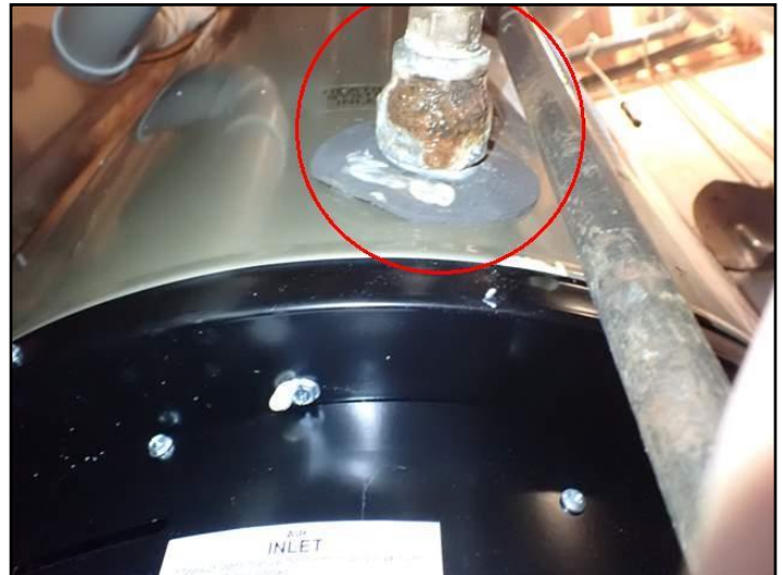
Leaky fitting on water heater
