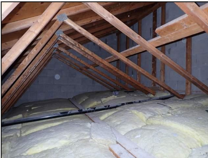
Insulation is evenly distributed
