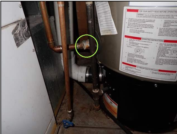
Leaky fitting on water heater
