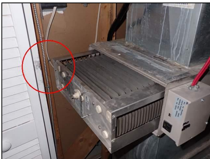
Door frame interferes with removal
