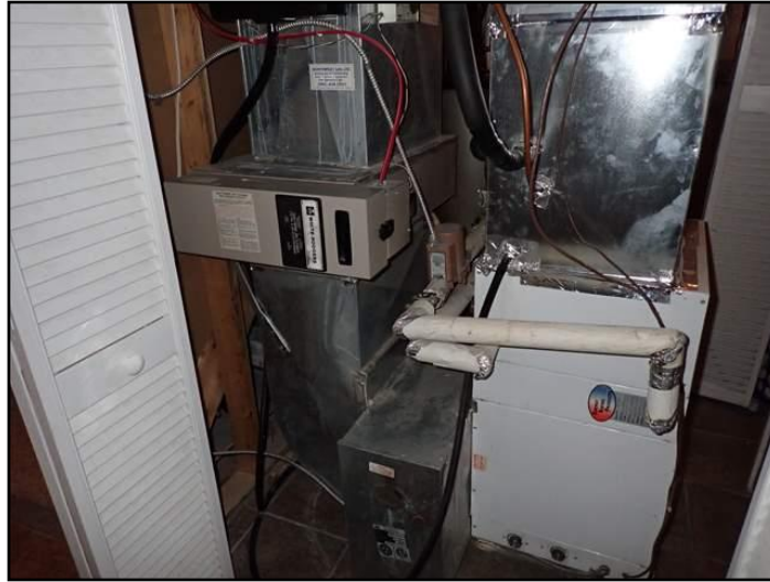
Combination heating system
