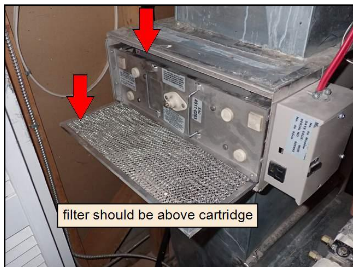
Improper orientation
