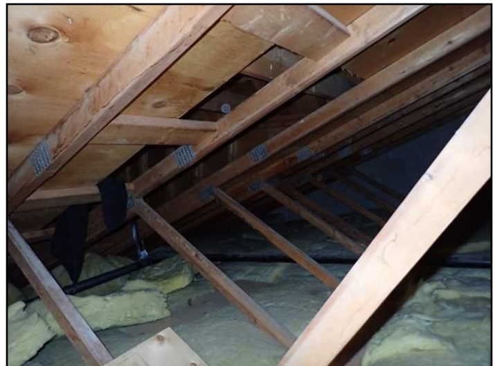
Insulation is evenly distributed
