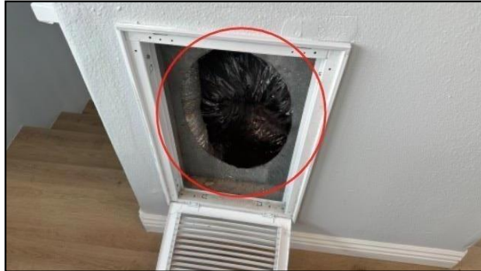
22. Poor arrangement- return duct
