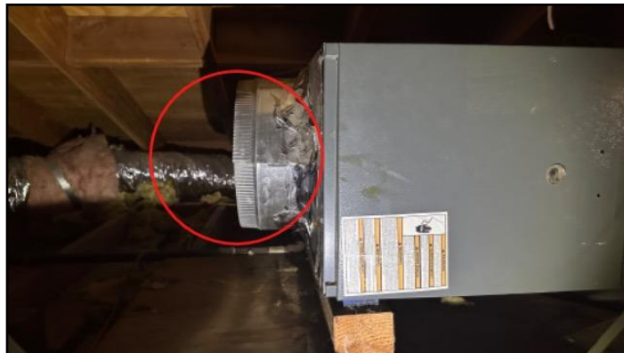
21. Missing return duct
