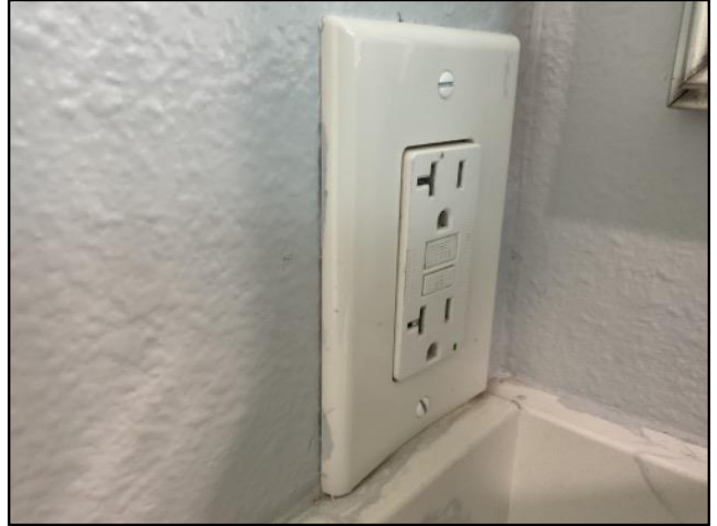
11. GFCI - master bathroom
