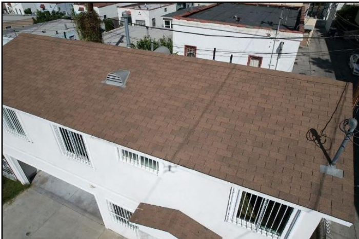
1. Asphalt shingles
