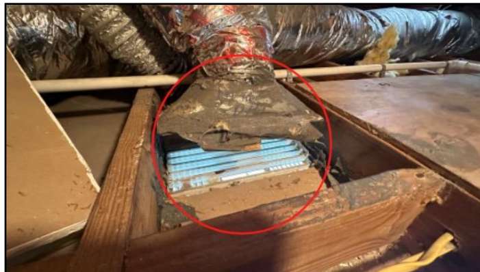
30. Damaged/Disconnected duct(s)
