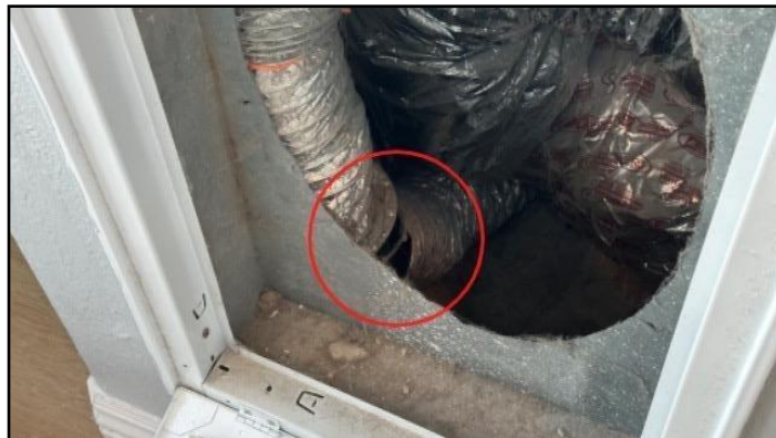
23. Damaged/Broken vent
