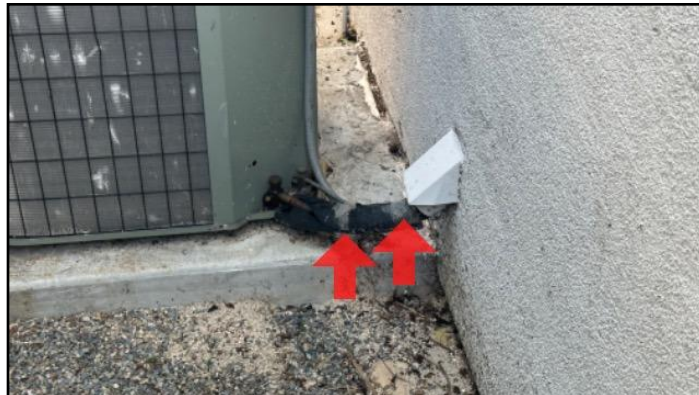
28. Damaged/Missing insulation
