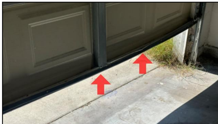
6. Damaged/Missing weatherstripping
