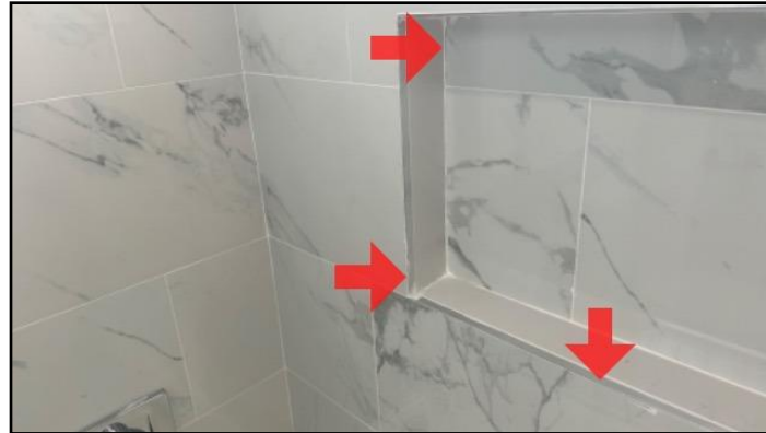
38. Damaged/Missing sealant
