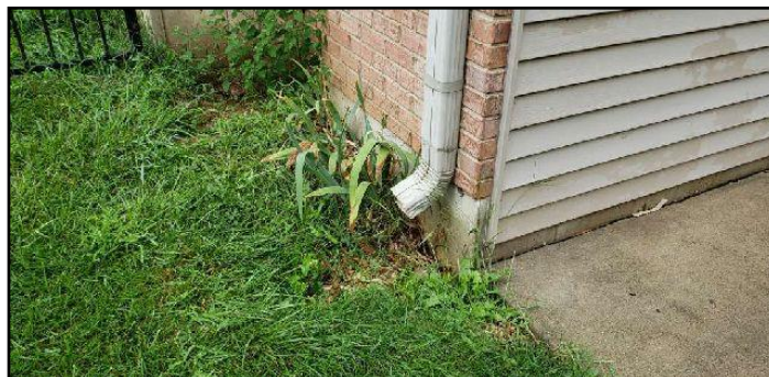
23. Should discharge 6 feet from building
