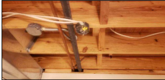
14. For junction box is missing
