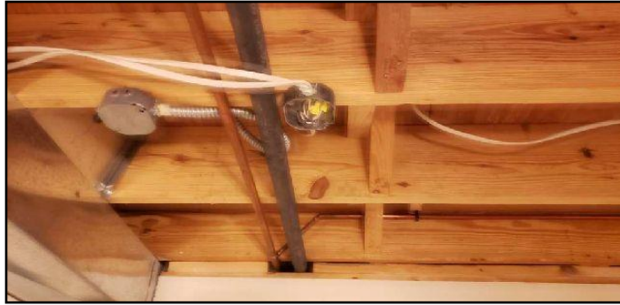
39. For junction box is missing
