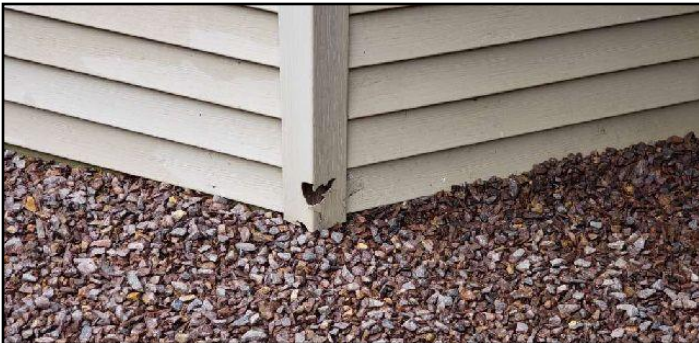
25. Mechanical damage
