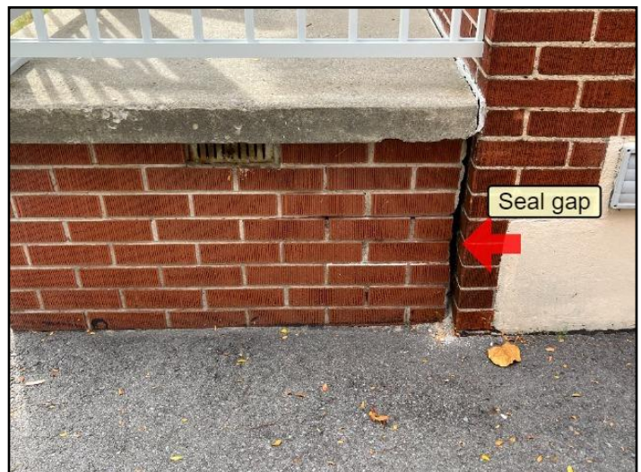
11. Gap where porch meets wall and mortar needed
