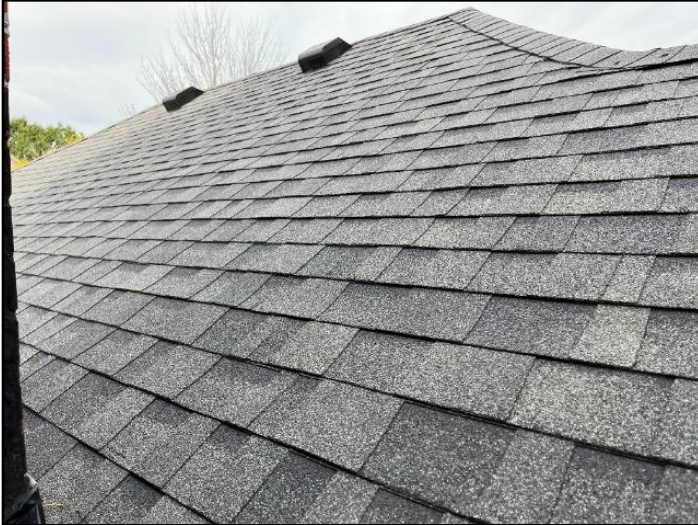
1. Asphalt shingles
