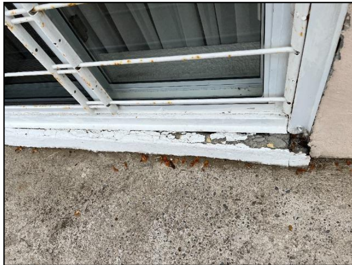
7. Sill deteriorated
