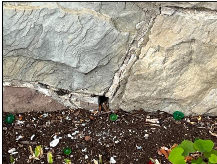
5. Mortar deterioration
