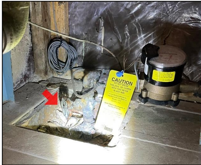
16. Main water shut off valve
