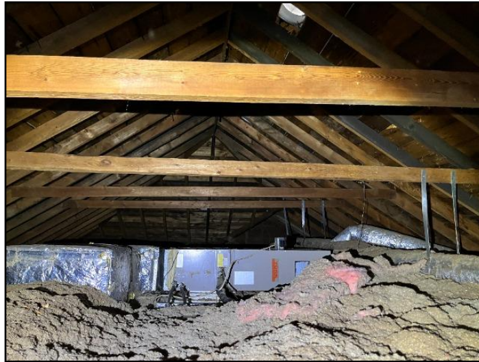
15. view of air handler and ducting in attic
