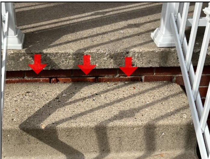
10. Spalling at brick riser
