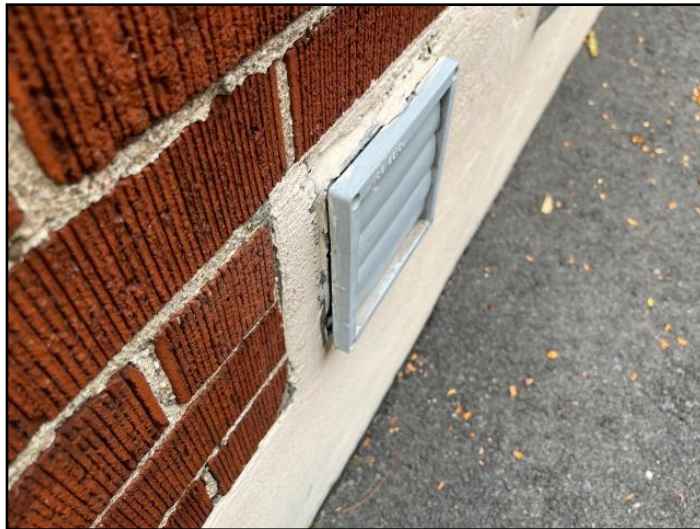
4. example caulking needed at vent
